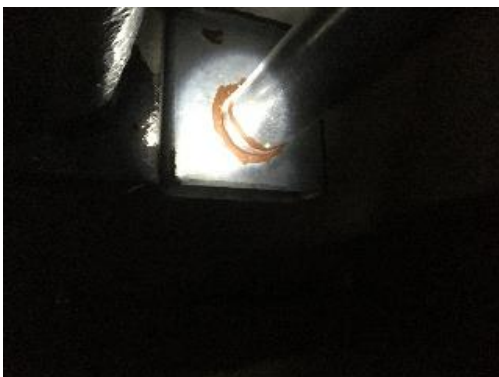
Photo 6: Non-asbestos brown mastic applied to joints of ductwork (Samples 0007A-C).
