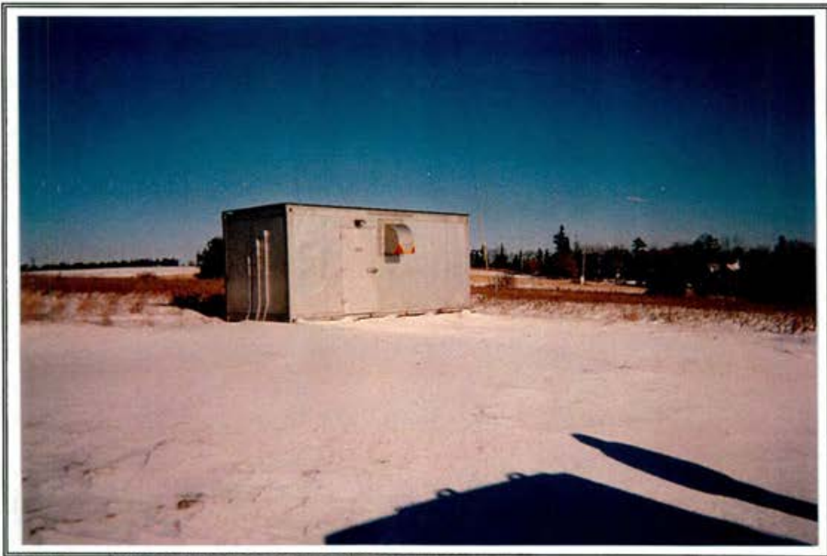
PHOTO 4: VIEW OF GENERATOR SHED LOOKING NORTHEAST.
