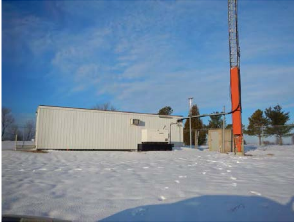
Figure 4: Cobourg MCTS Shelter
