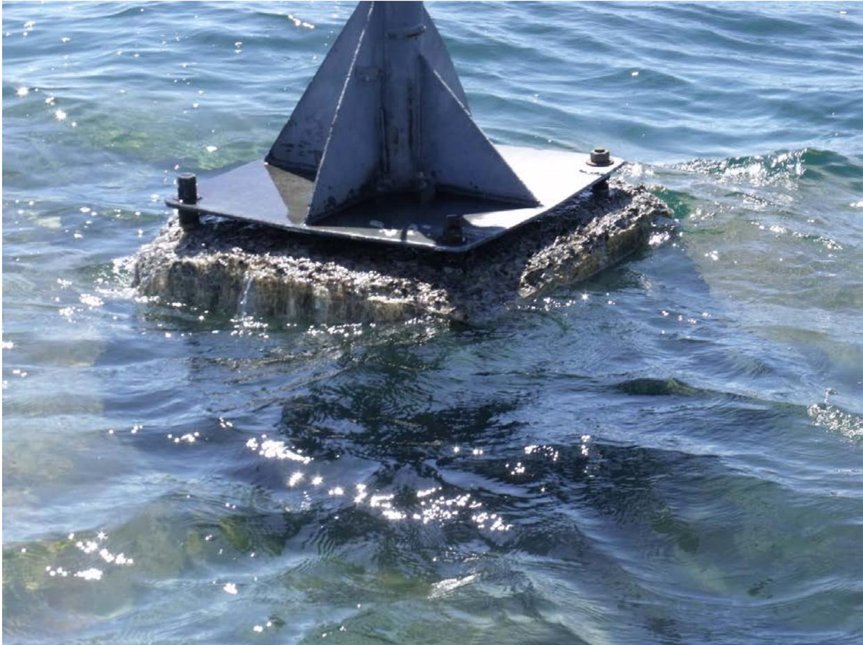
Figure 7 – Existing weathered pier (to be removed)
