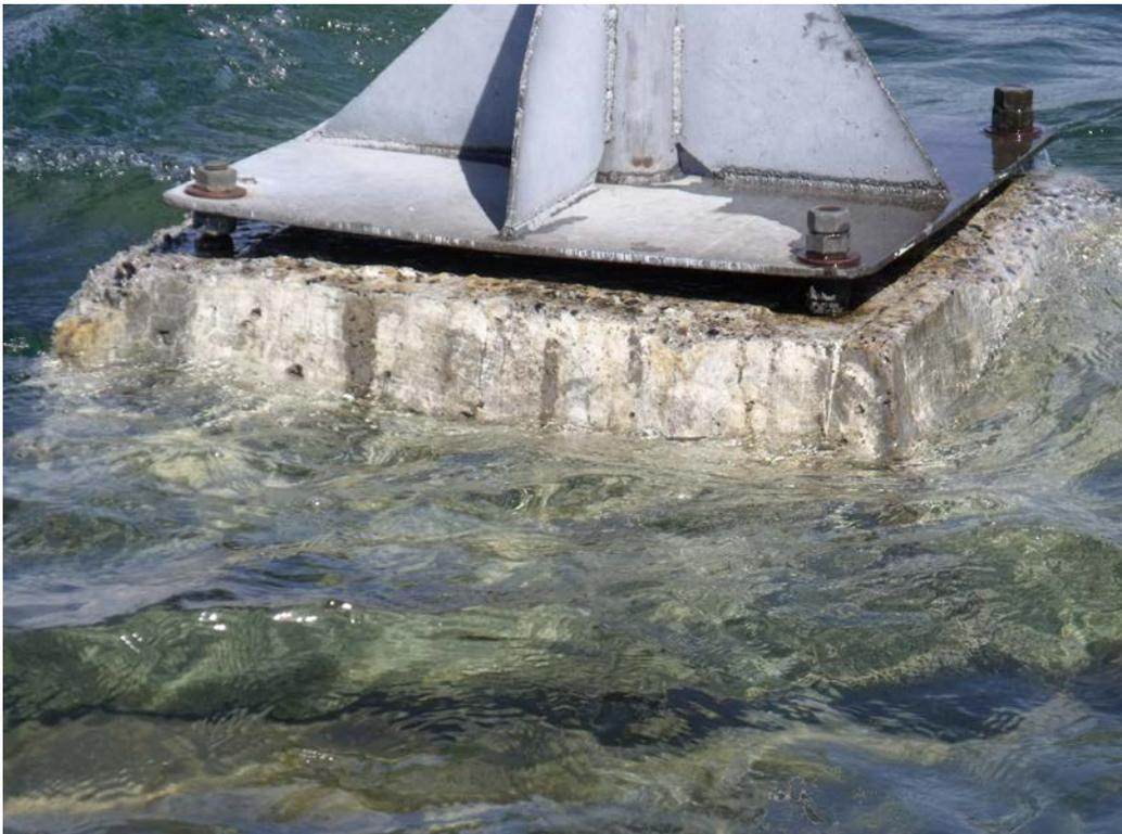
Figure 6 – Existing weathered pier (to be removed)
