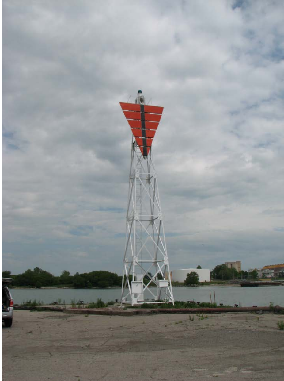
Figure 7: Existing Tower to be demolished
