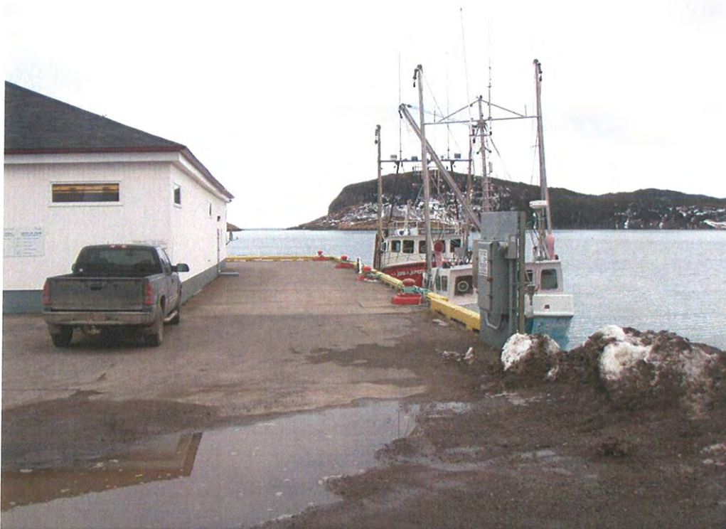
Photo 10: Standing water observed in asphalt parking area, looking southeast.
