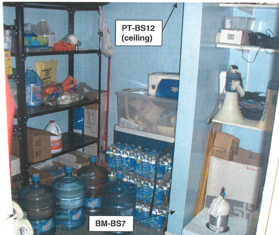
Photo 12: Beige floor tile in Storage Area.
