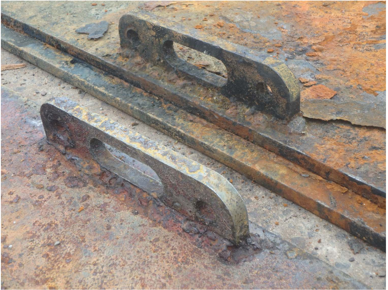
Access Door – 13 mm plates to be cut
