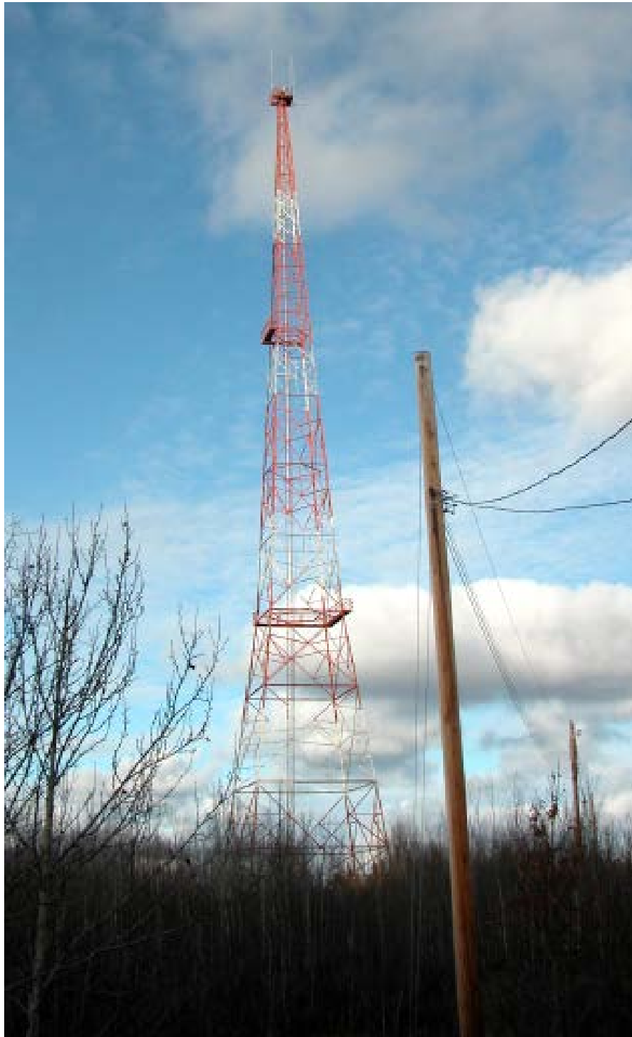
Existing tower to remove
