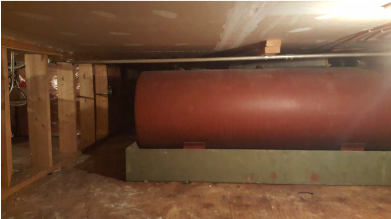
Photo 15 Interior Tanks to be removed
