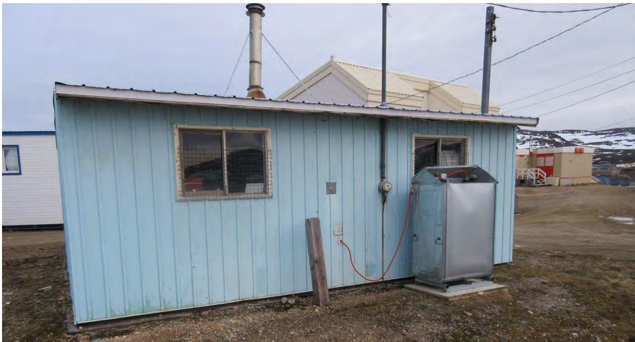
Photo 6 Rear Elevation of Fuel Tank
