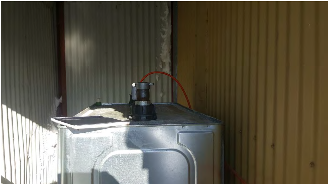
Photo 8 Tank in Side Shed
