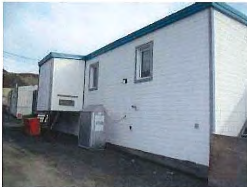
Photo 1: Outdoor above ground fuel tank
