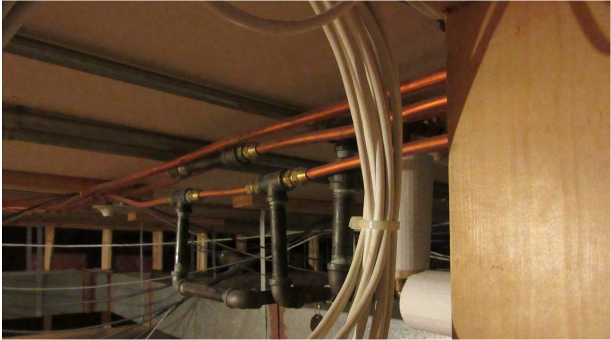
Photo 15 Crawl Space Piping
