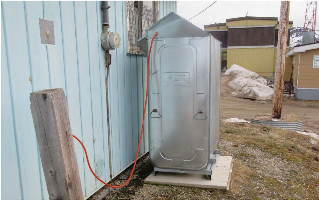
Photo 7 Fuel Tank Exterior
