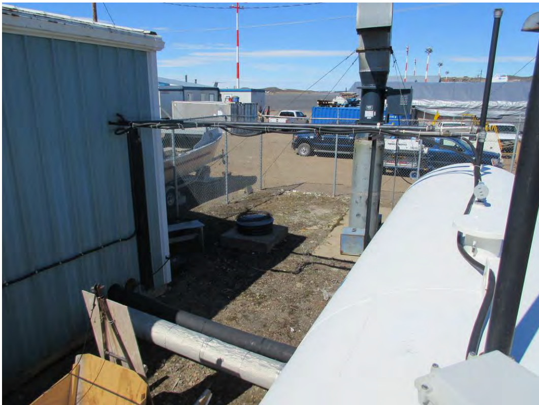
Photo 2 Top of Tank
