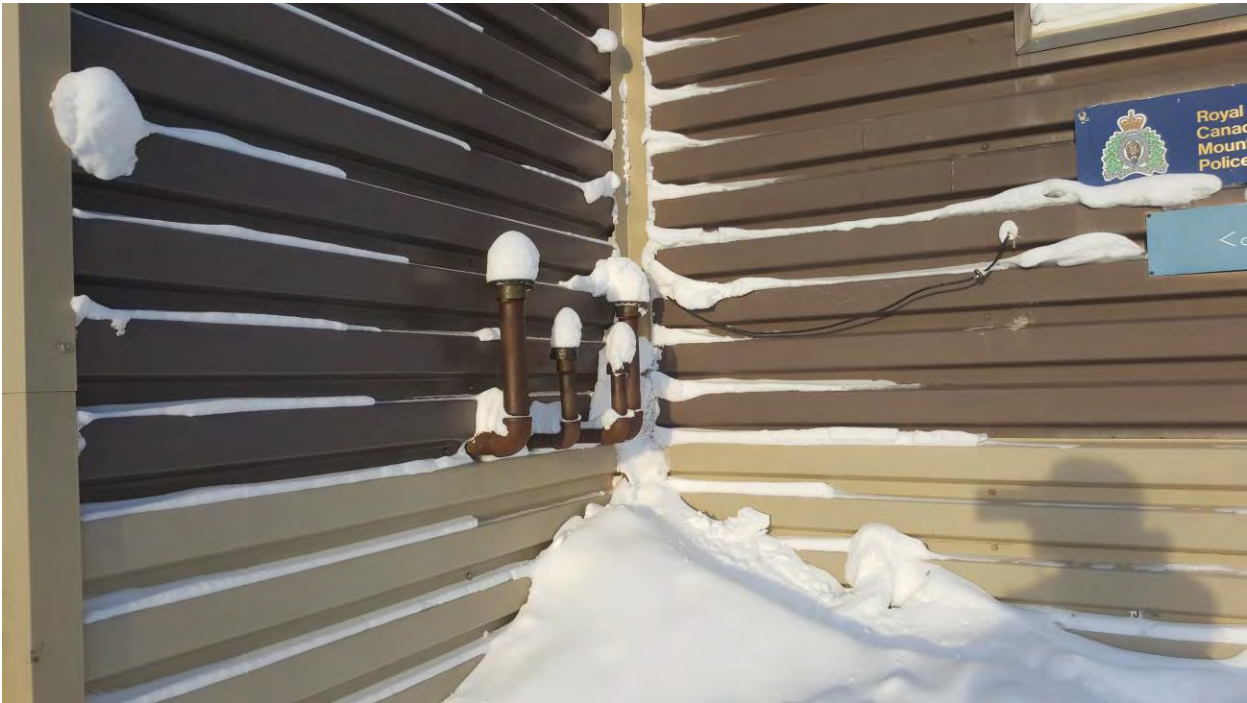
Photo 13 Exterior Fill and Vents
