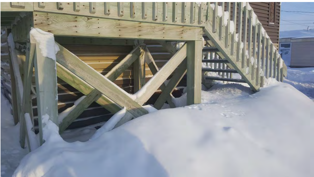
Photo 14 Exterior Stairs to be Removed and Re-Installed
