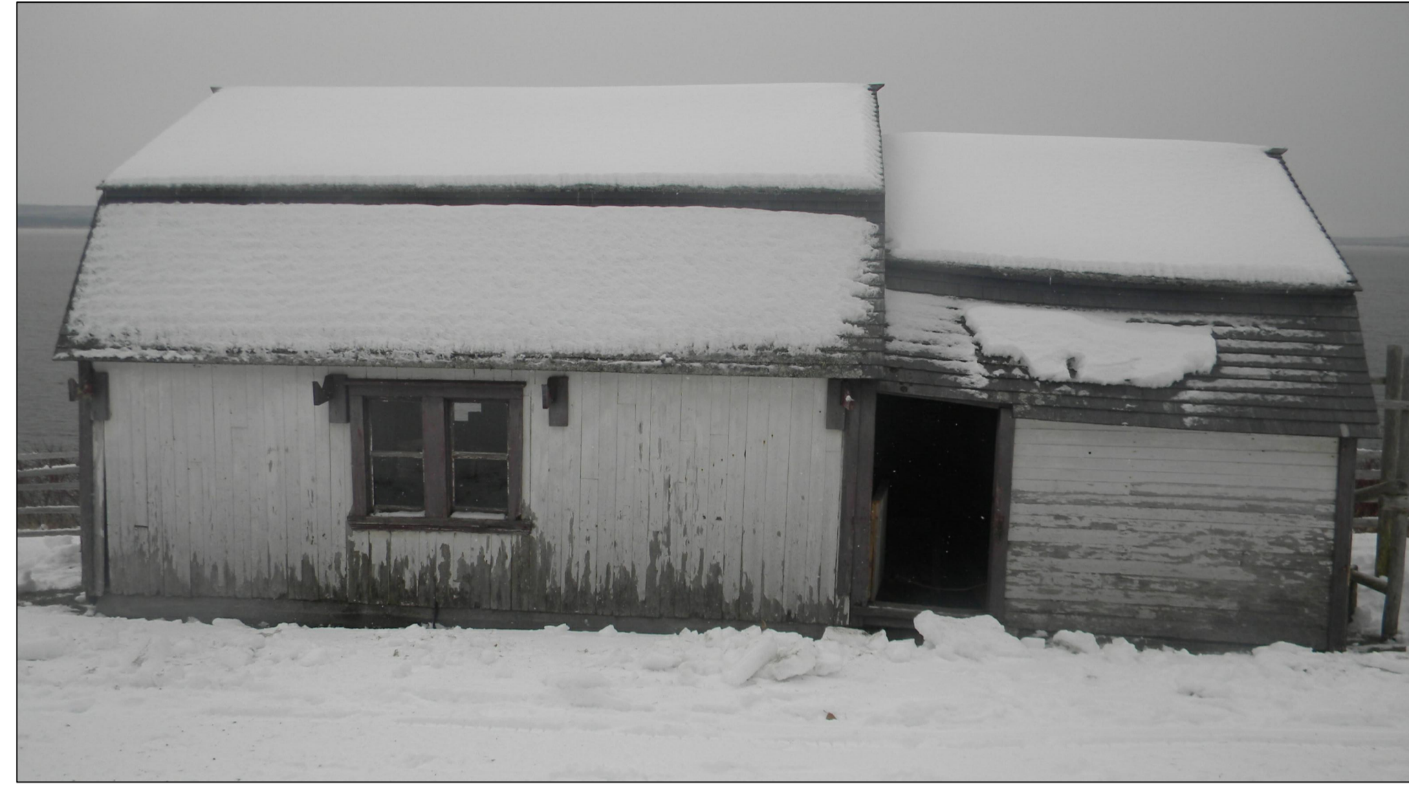
EAST ELEVATION - PHOTO
