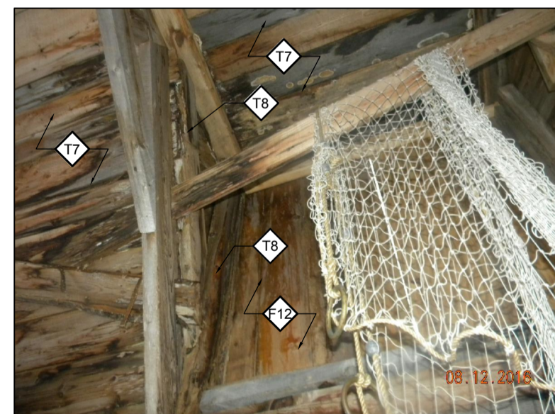
PHOTO 4 - ROOF SUPPORT BOARD AND FRAME TO REPLACE AROUND THE WINDOW DORMER.
