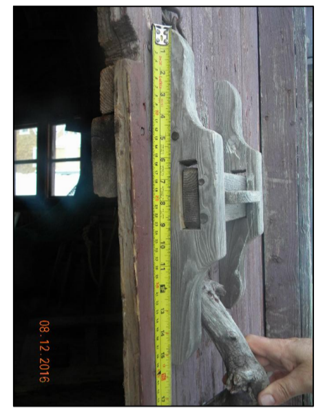
PHOTO NO.1: HANDLE AND SLIDING LOCK SYSTEM FISH HANGAR DOOR
