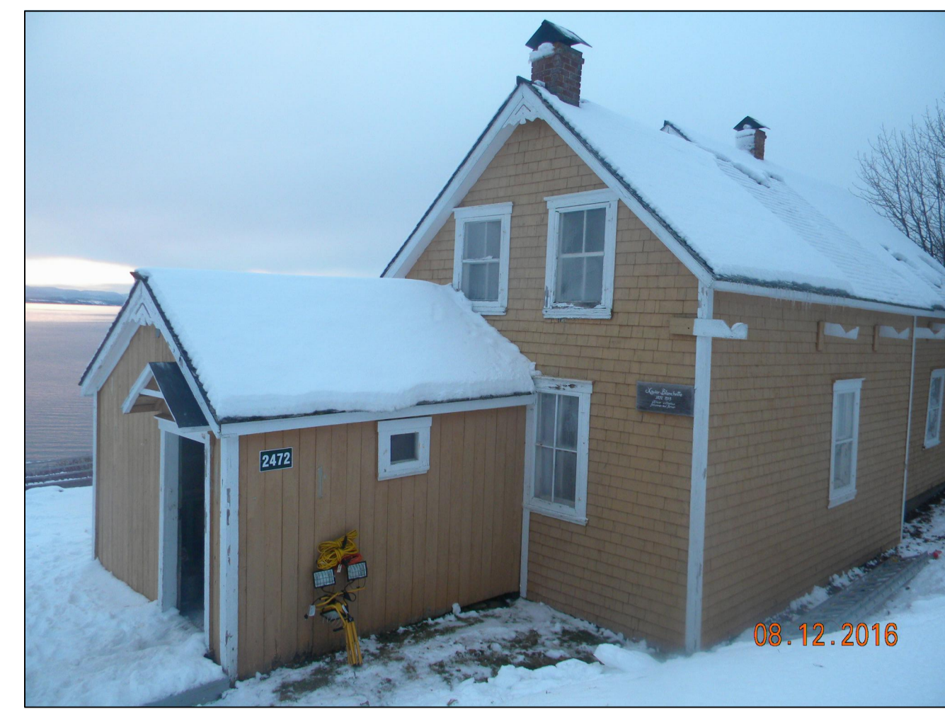
RIGHT ELEVATION - PHOTO
