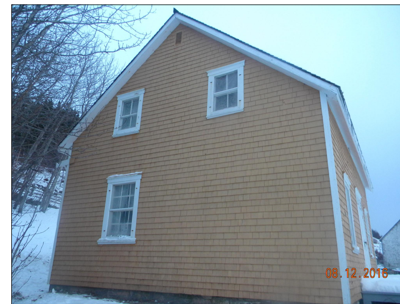
LEFT ELEVATION - PHOTO
