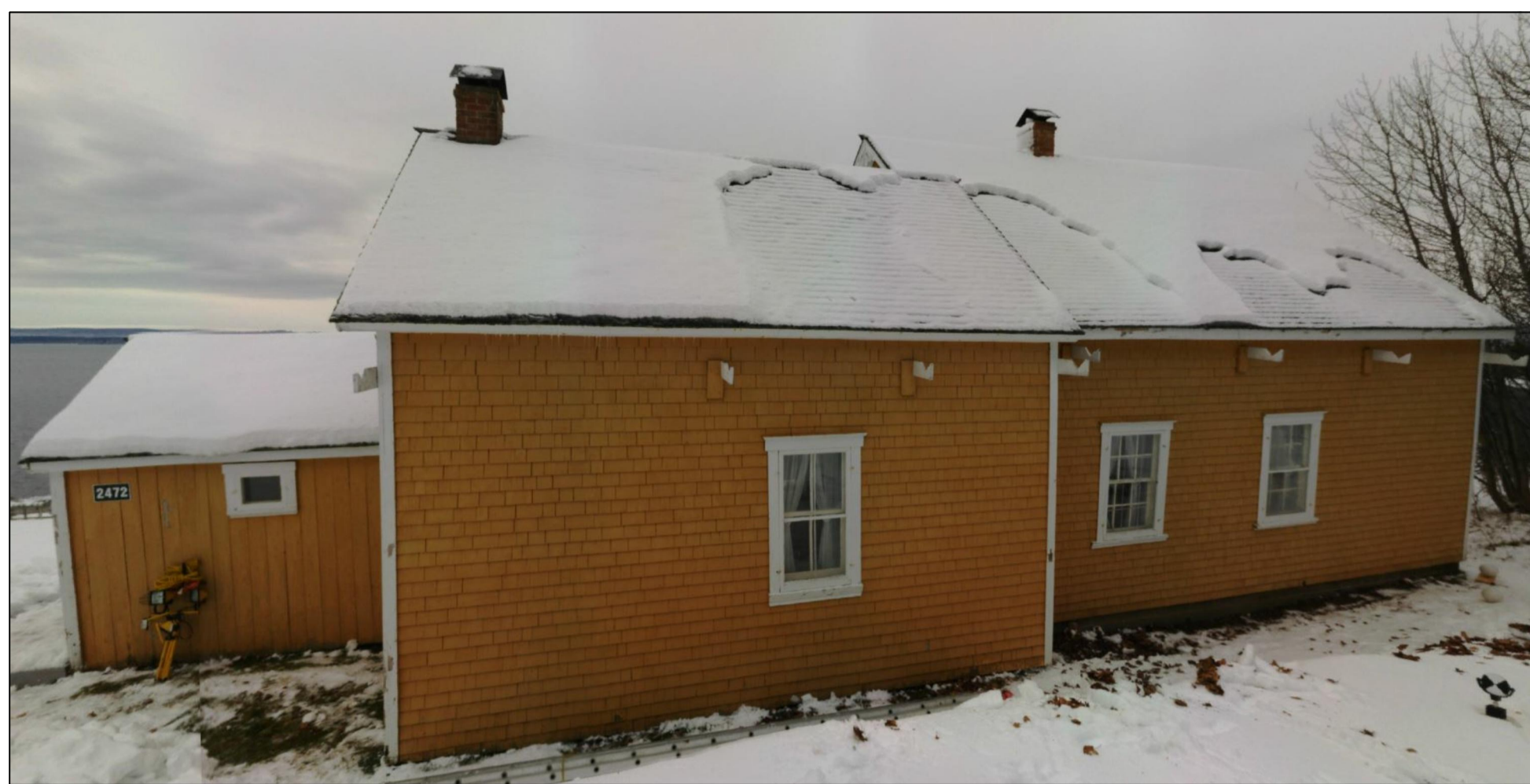
BACK ELEVATION - PHOTO
