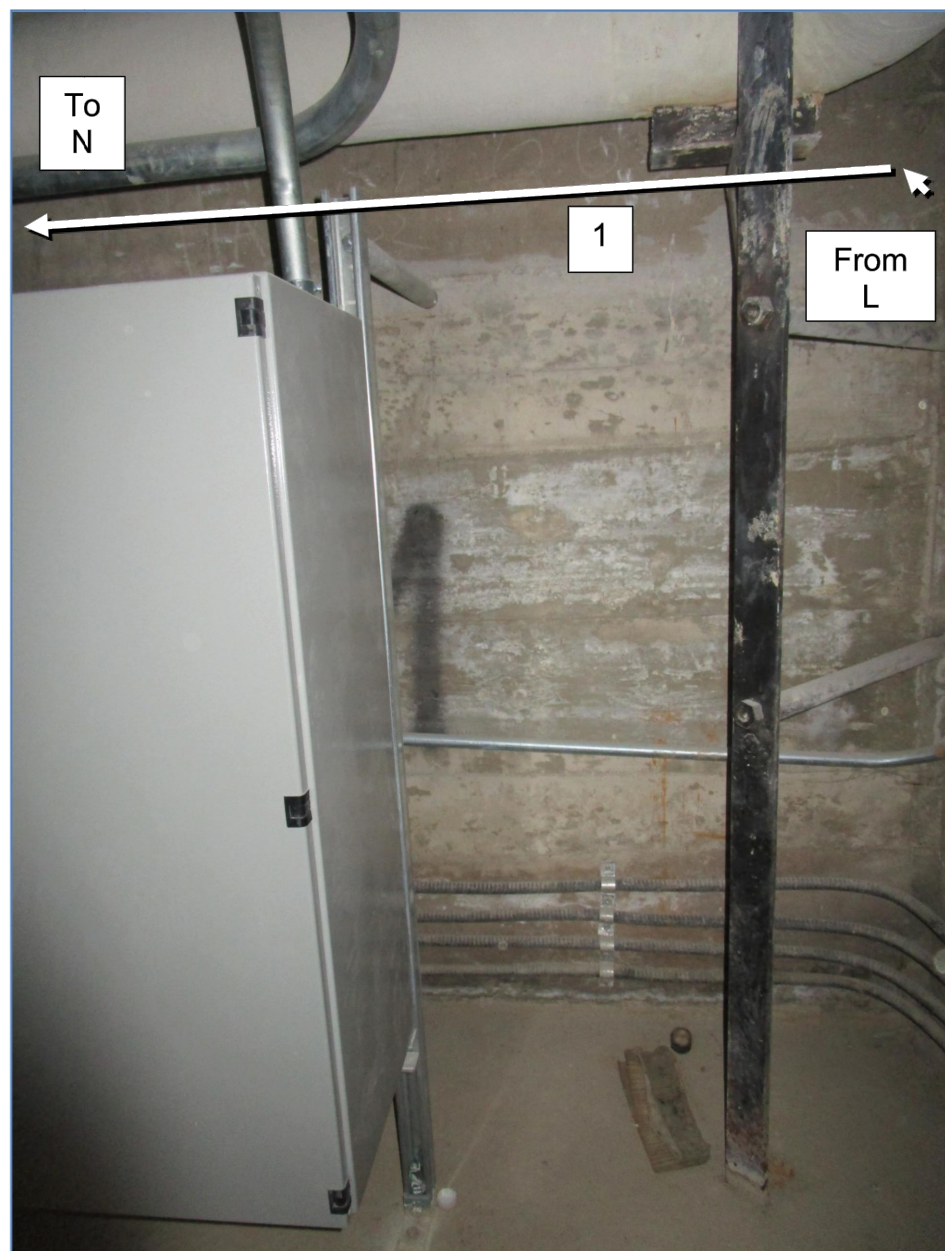
Figure 15 - Location M, conduit crossing above existing junction box JB-G (View 1)
