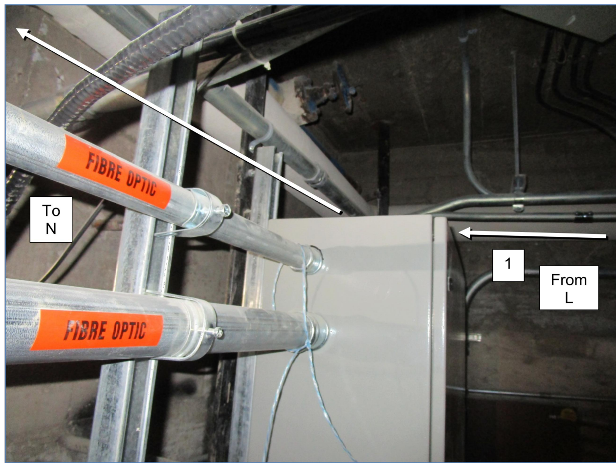
Figure 16 - Location M, conduit passing over existing junction box JB-G (View 2)
