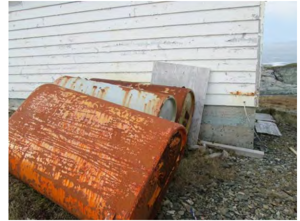
Photo 141: View of abandoned ASTs on-Site.
