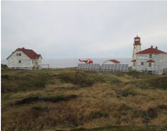
Photo 1: View of the Belle Isle North Lightstation located on Belle Isle, NL.
