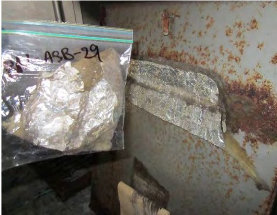
Photo 31: View of grey fibreglass insulation sample BN-ASB-29.
