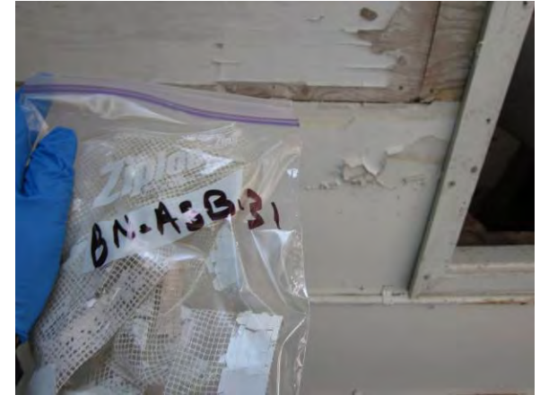
Photo 33: View of drywall joint compound sample BN-ASB-31.
