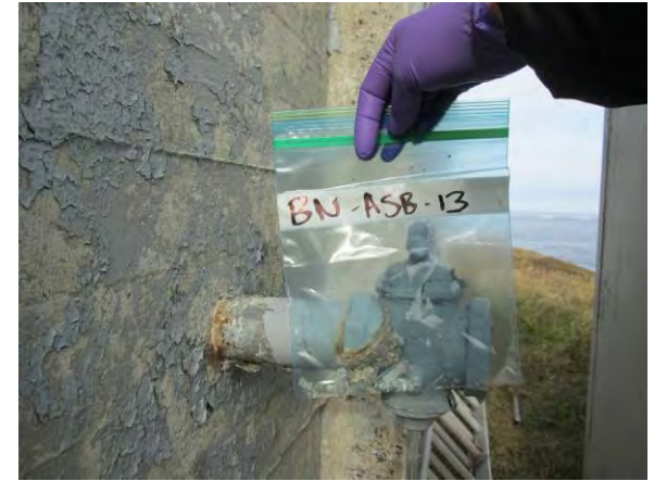
Photo 15: View of light grey caulking sample BN-ASB-13.
