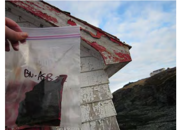
Photo 39: View of red asphalt shingle with paper/felt backing sample BN-ASB-37.
