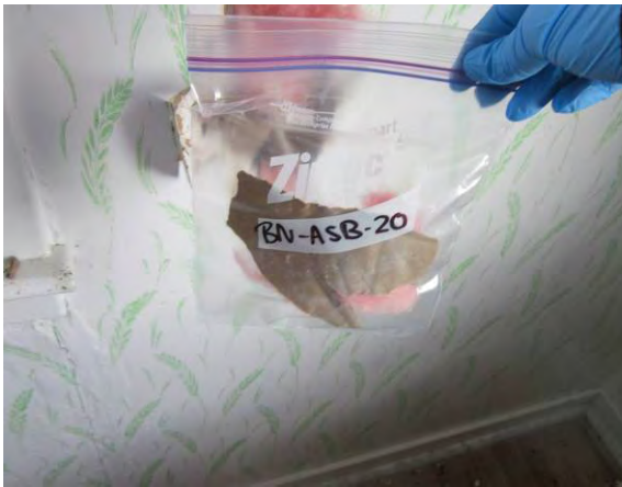
Photo 22: View of pink fiberglass insulation with paper backing sample BN-ASB-20.
