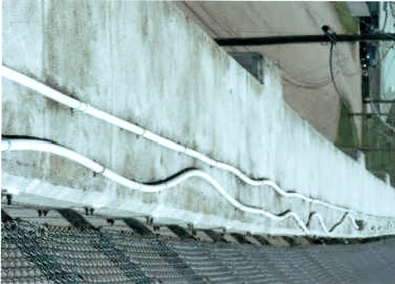
B – BETWEEN TOWER D2 / D3 TWISTED CONDUITS
