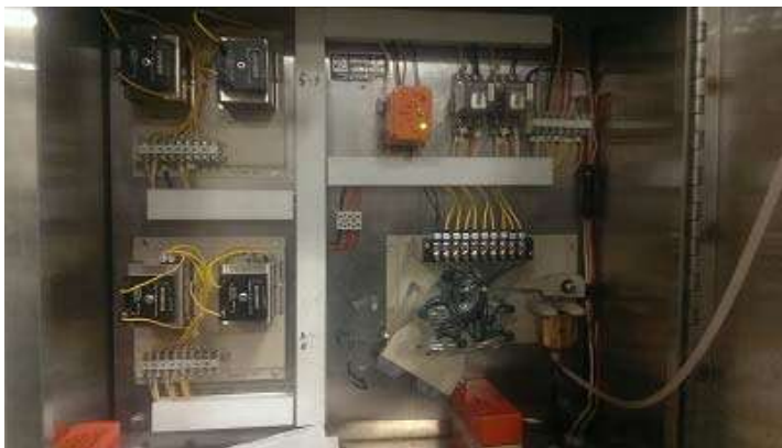
Water tower controls, alternating pump switch, mercury filled contact
