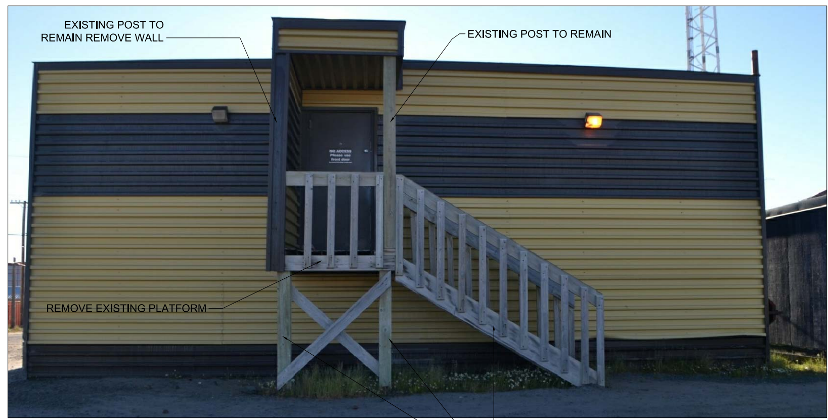
2 EXISTING STAIR ELEVATION A0.1 SCALE: NTS
