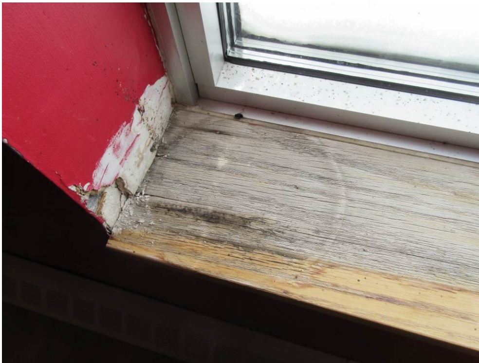
Photo 12 Existing Window Sill
