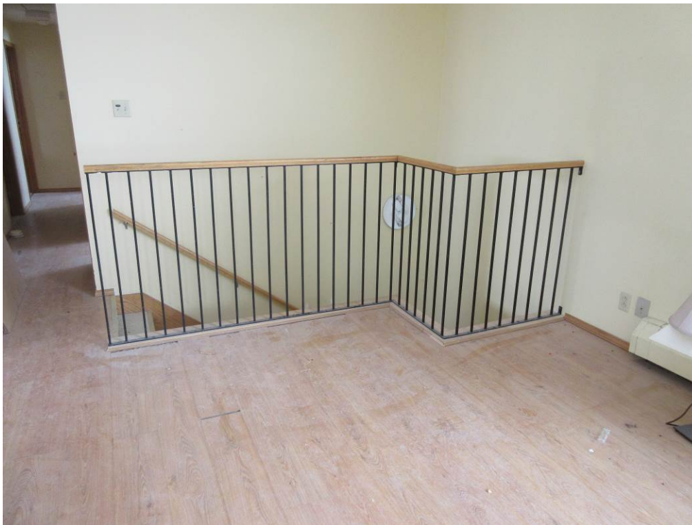
Photo 10 Existing hand rail to be removed
