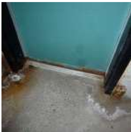
March 2016. Note rusting at base of steel door in parking garage.
