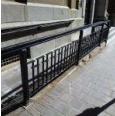
March 2016. Deterioration at ramp due to salts/ winter conditions.
