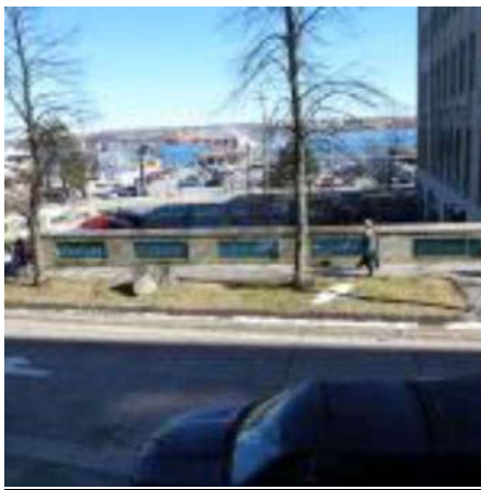
March 2016. Note granite stone portion of concrete reinforced retaining wall that occurs between the exterior parking area and Bedford Row.
