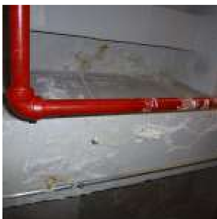
March 2016 Water entry at ceiling in Elevator machine Room in Tower.
