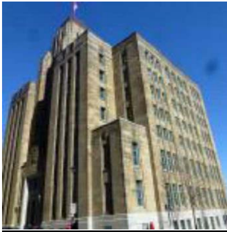
March 2016. Limestone Masonry blocks of main building (fls1-7) and tower as well as granite blocks of base (basement level).
