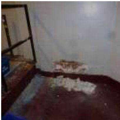
March 2016 Plaster blow out in Tower Elevator machine Room from water entry.
