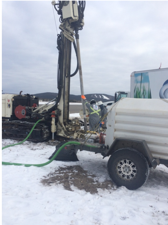
Photograph 3: Sonic drilling at APEC 22 E.
