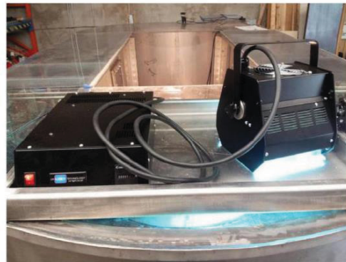
Figure 5. Ultra Violet Light mounted above Access Port.
