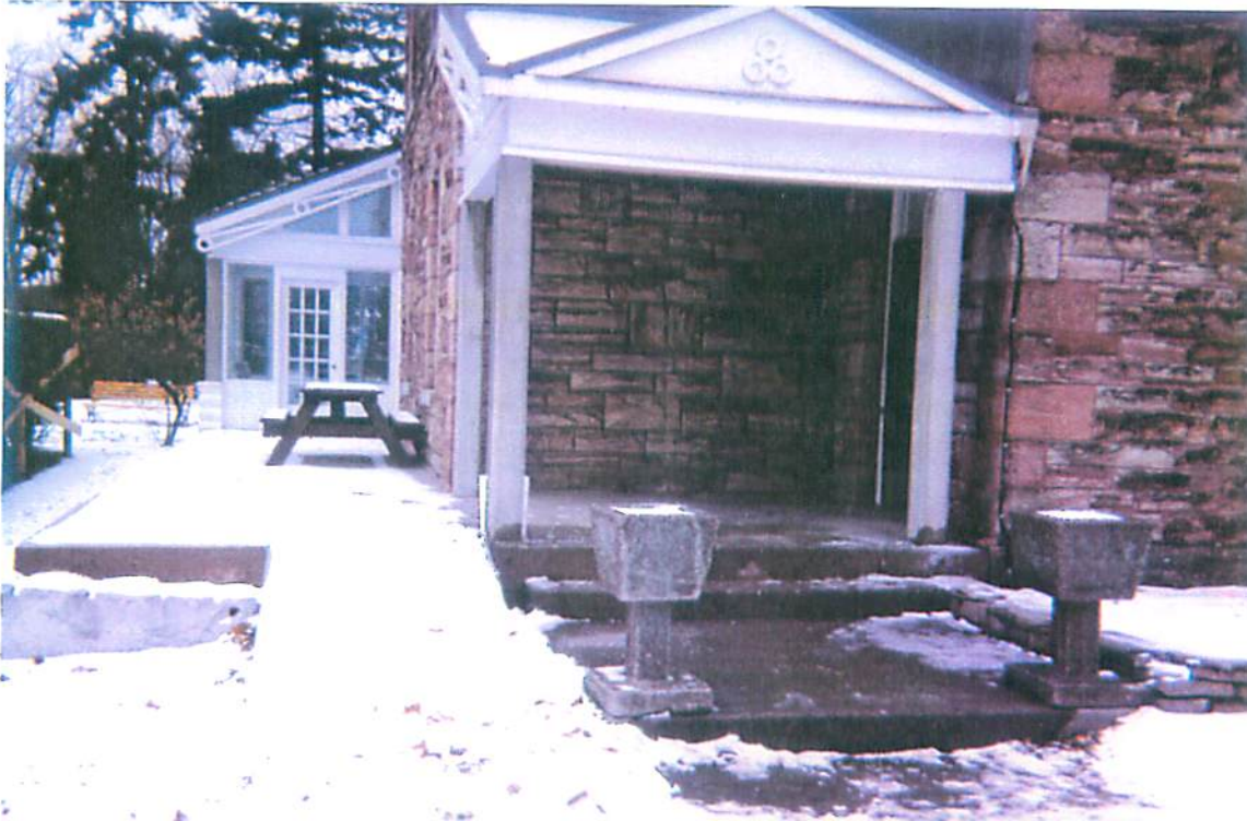
PHOTOGRAPH #4 The Main Entrance
