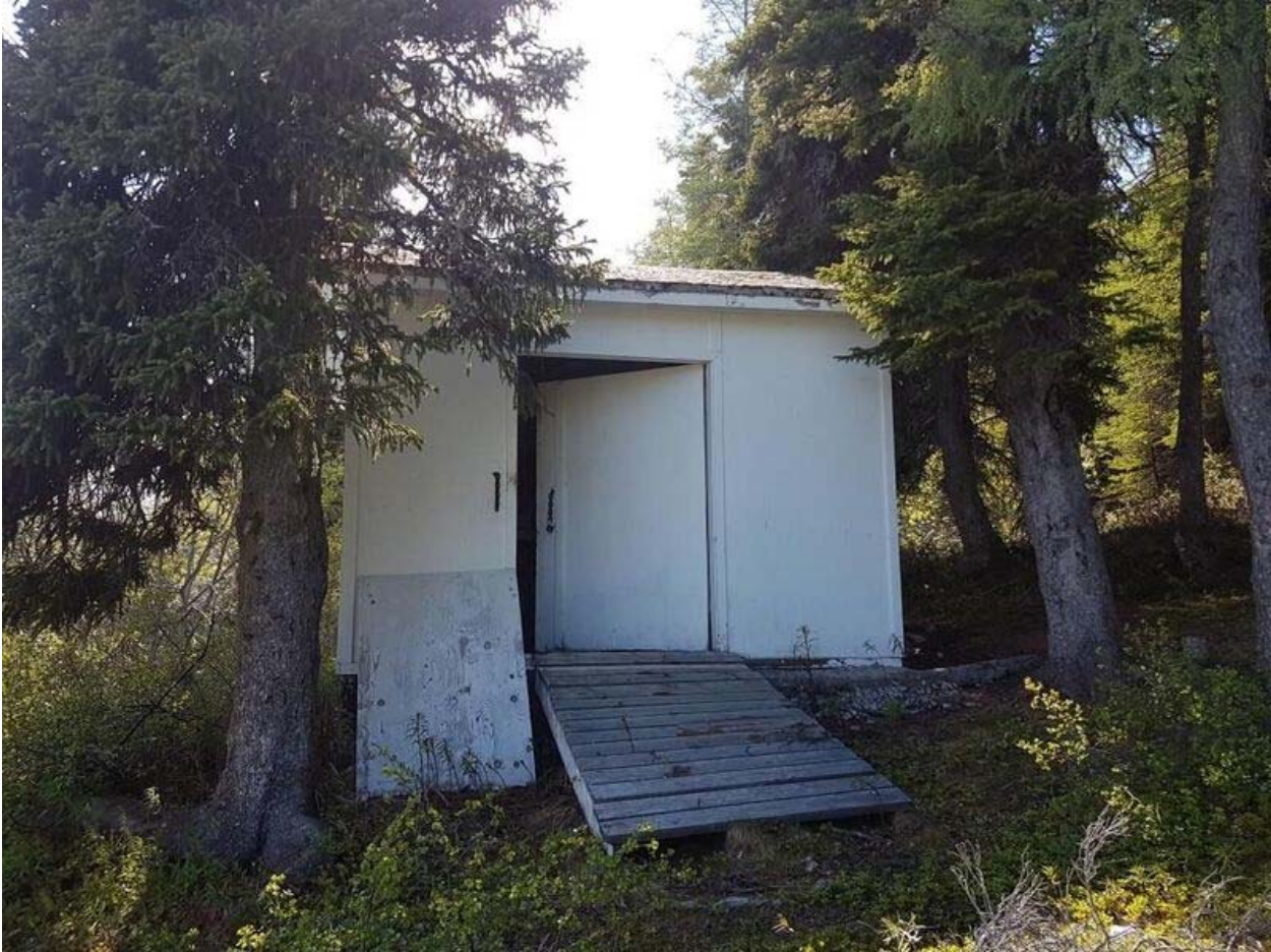
General view - shed
