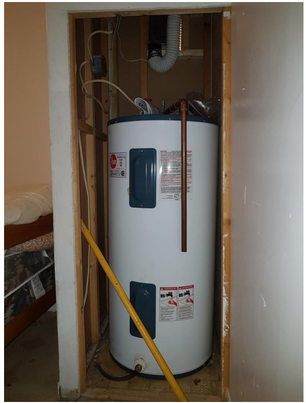
Photo 56 – Trailer, Bedroom #1 HWT
