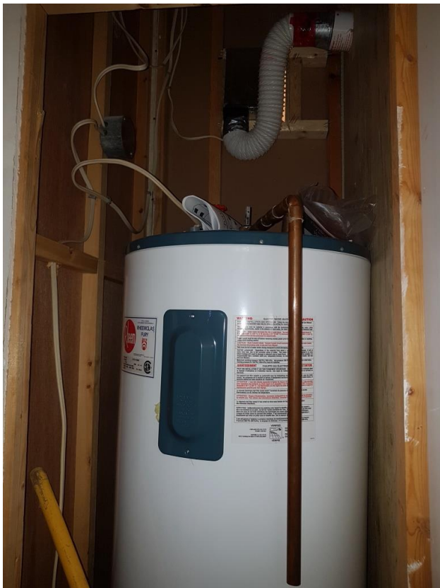
Photo 57 – Trailer, Bedroom #1 HWT
