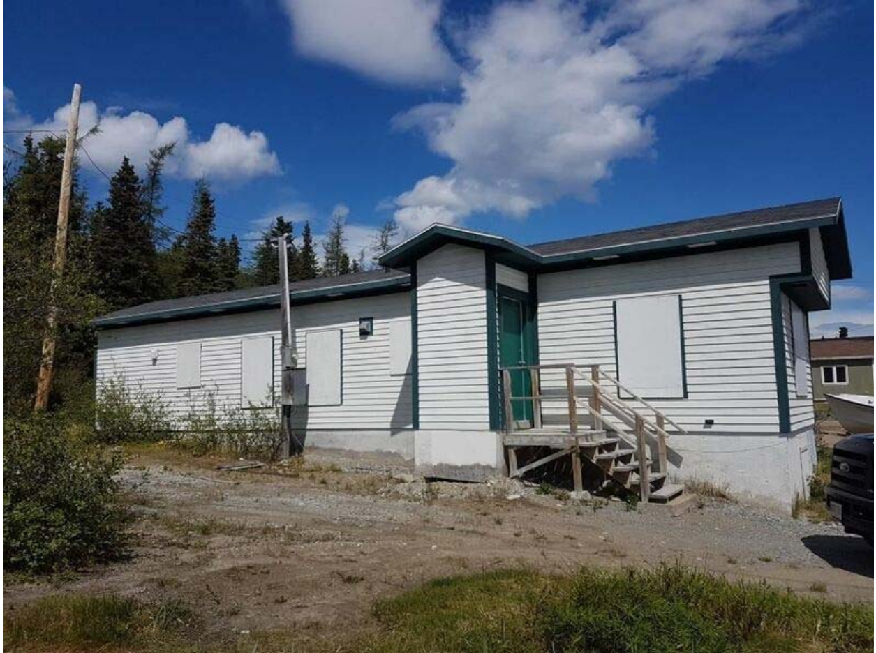
General view - trailer
