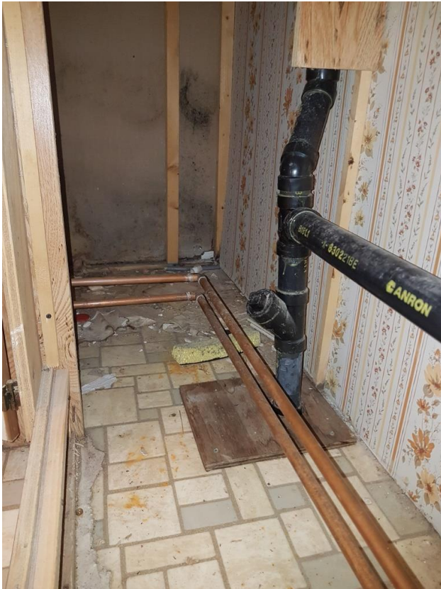
Photo 65 – Trailer, Bathroom, Plumbing Under Vanity and Bathroom Storage Closet
