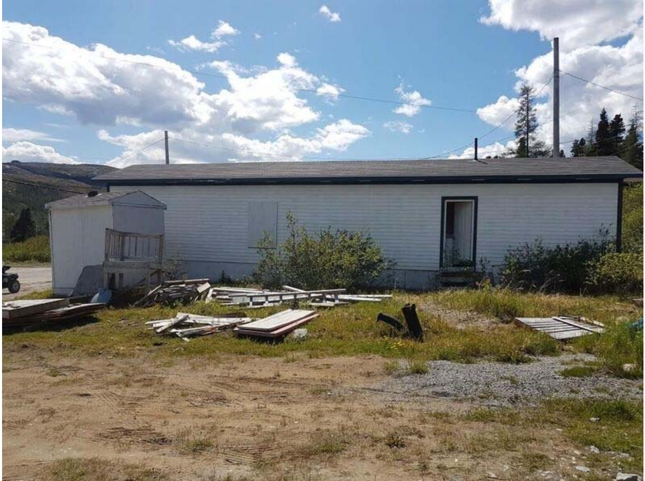
General view - trailer
