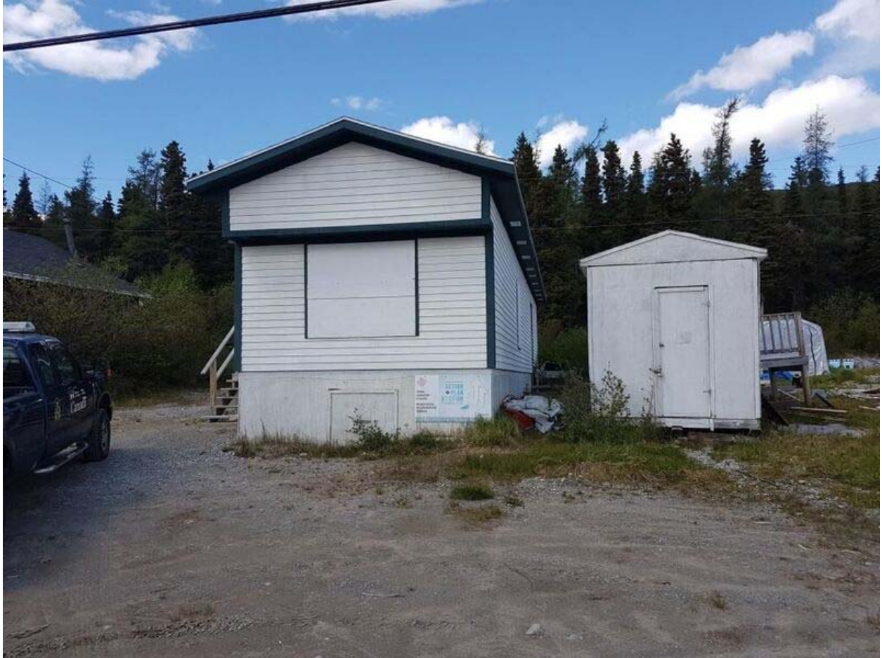
General view - trailer
