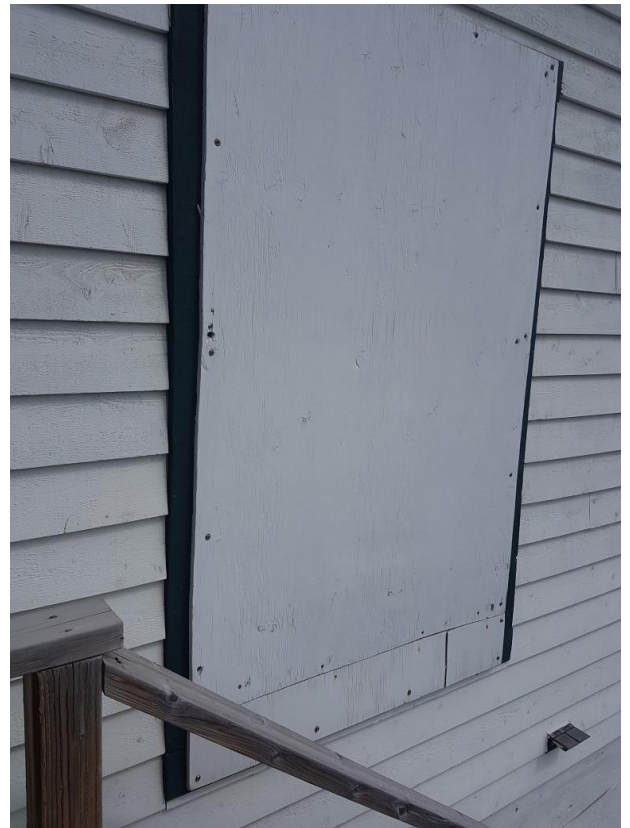
Photo 14 – Trailer, Typical Plywood Cover Over Windows
