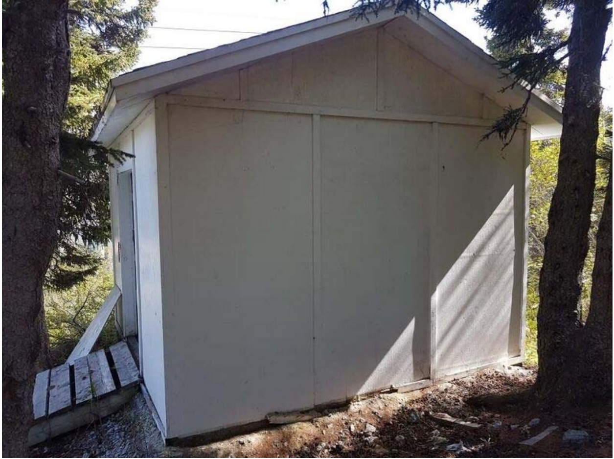
General view - shed
