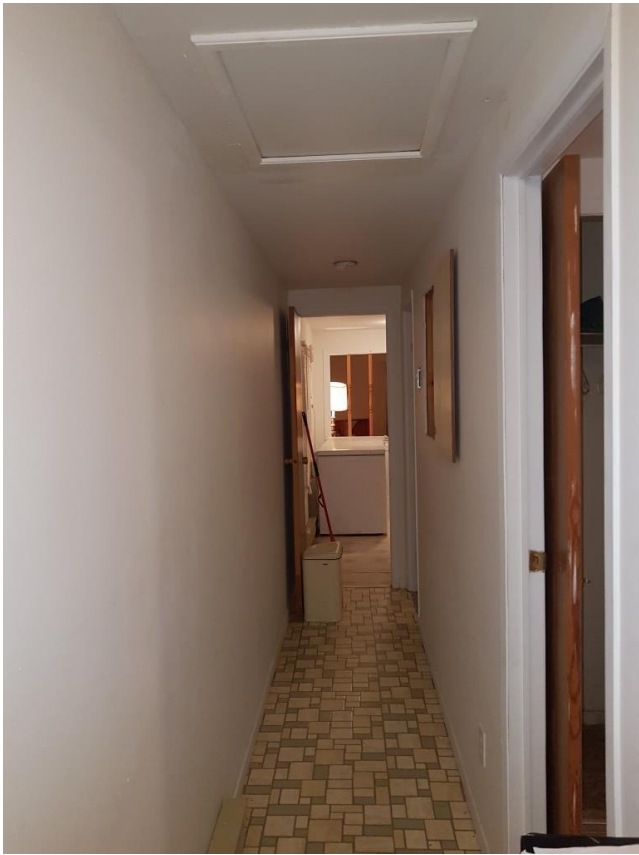
Photo 39 – Trailer, Hallway, View from Bedroom #1
