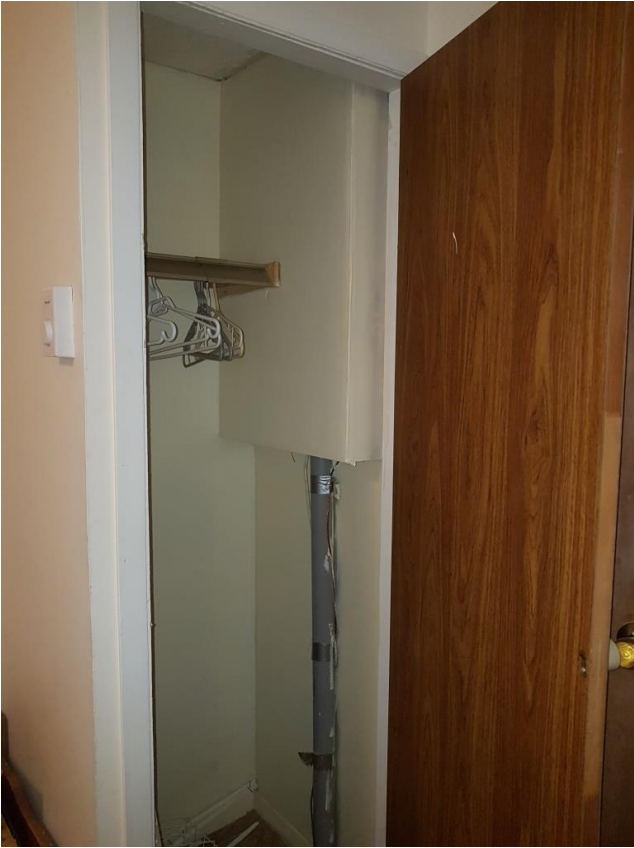
Photo 47 – Trailer, Bedroom #3 Closet (Note electrical conduit and box-out for panel)
