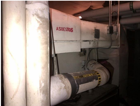
Insulation contains Asbestos
