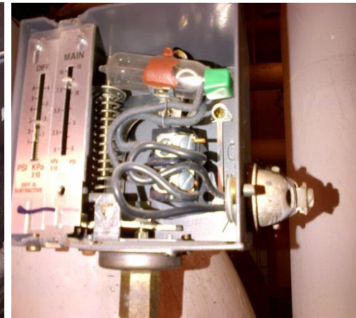
Mercury Switches on heating systems mechanical room
