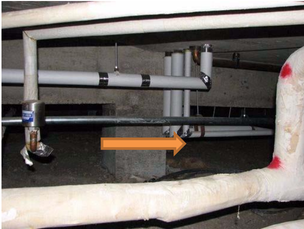
Asbestos containing piping (Red Dots) inside the crawlspace. (Confined Space)
