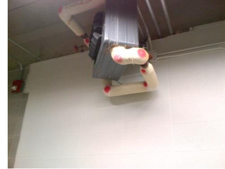
Asbestos Pipe Insulation
