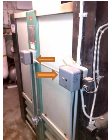
Mercury Switches on heating systems mechanical room
