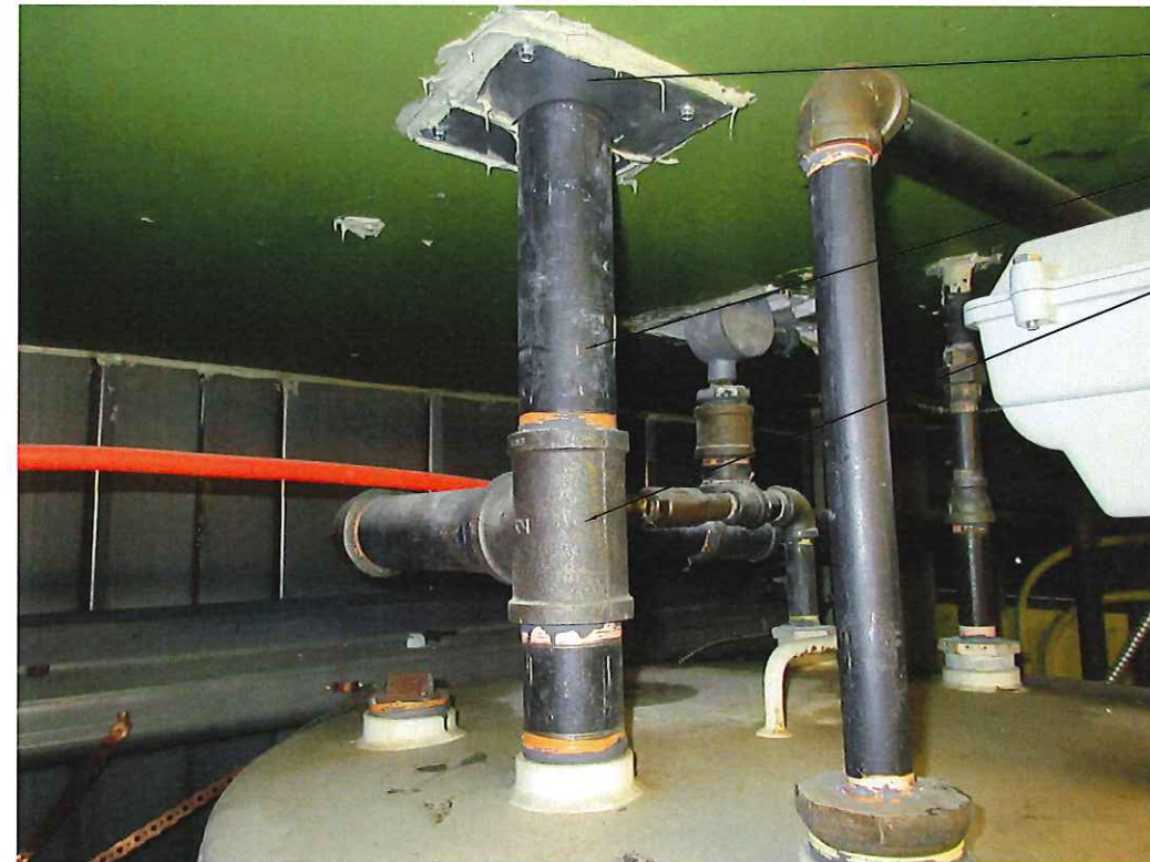
2 VENT ON TOP OF AUXILARY TANK M1.1 SCALE: NTS
