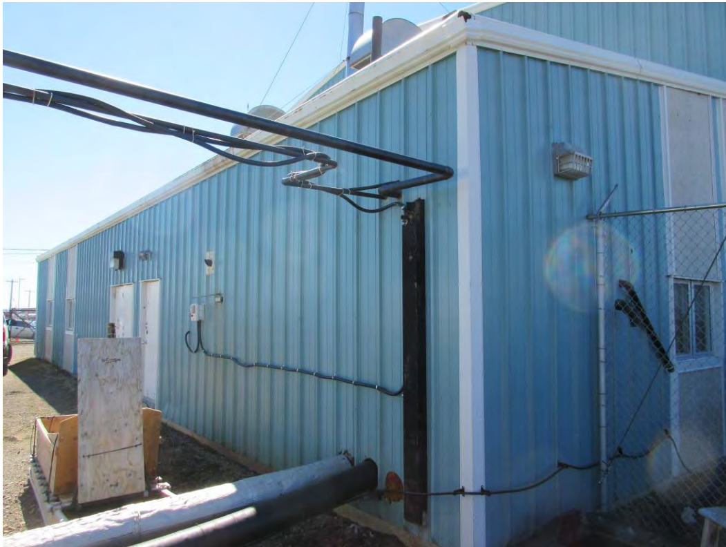
Photo 4 Piping into Building
