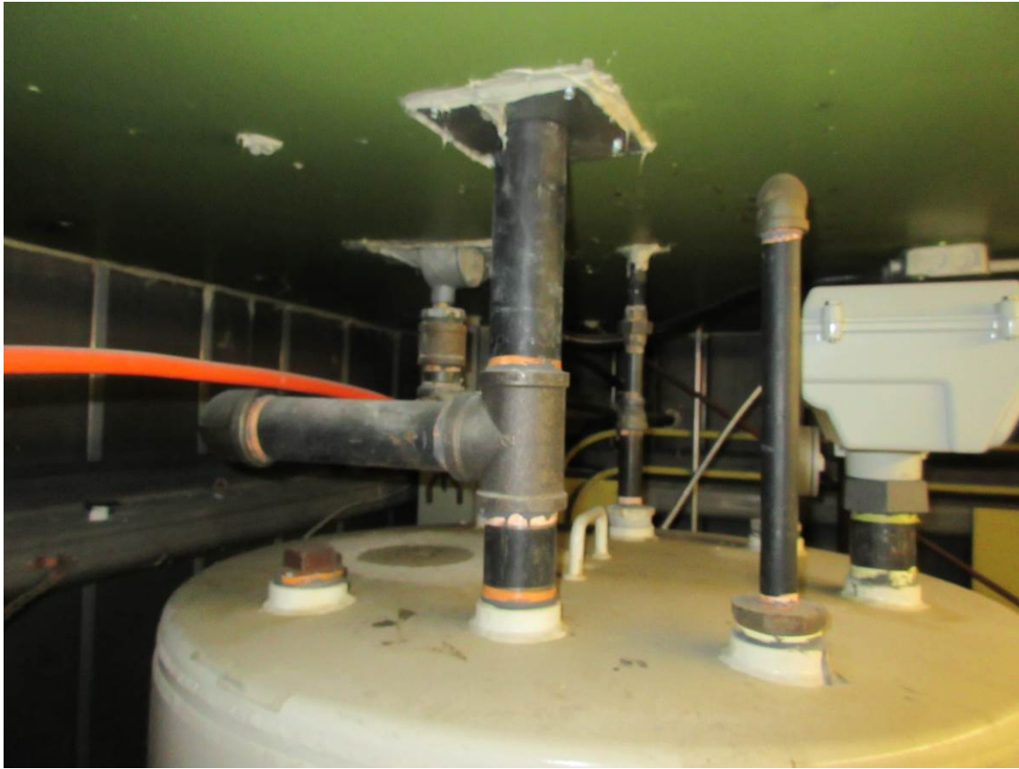
Photo 7 Vent Through Roof
