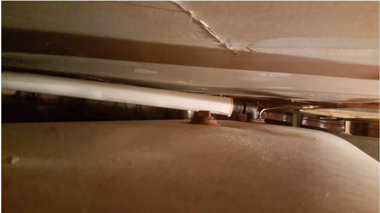
Photo 17 Interior Venting to be removed
