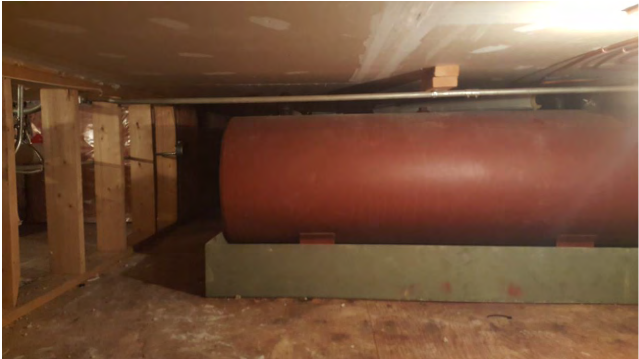
Photo 15 Interior Tanks to be removed
