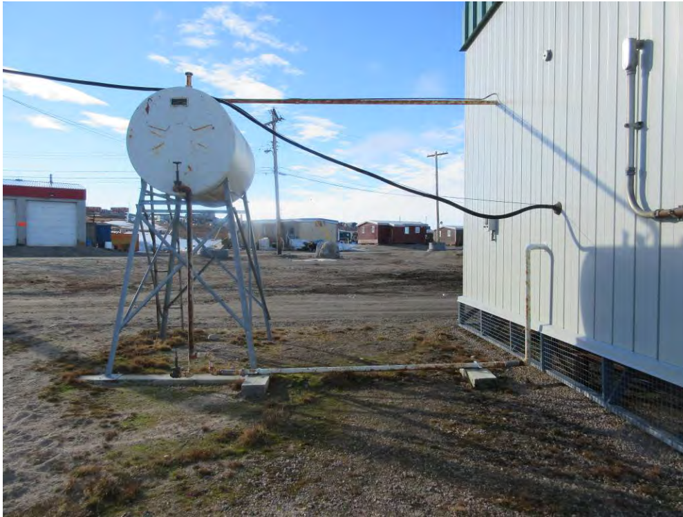
Photo 11 Exterior Tank Elevation
