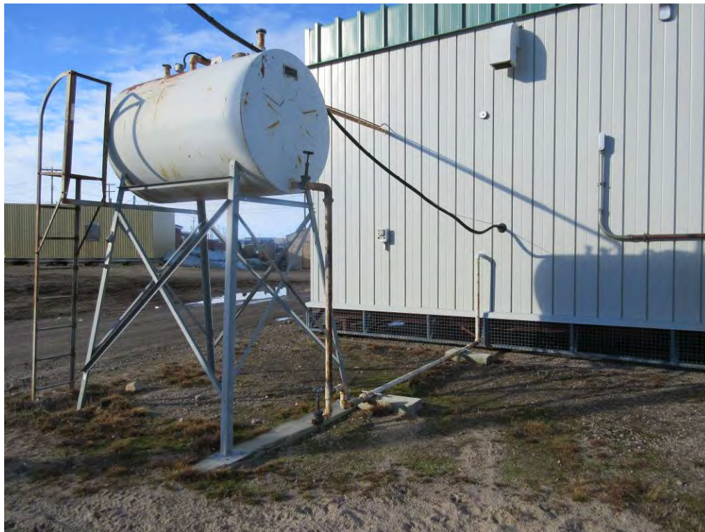
Photo 10 Exterior Tank Elevation
