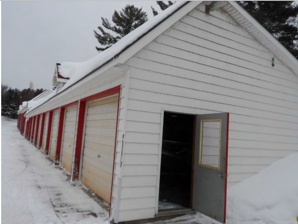
Photo 7: Storage Buildings (east).
