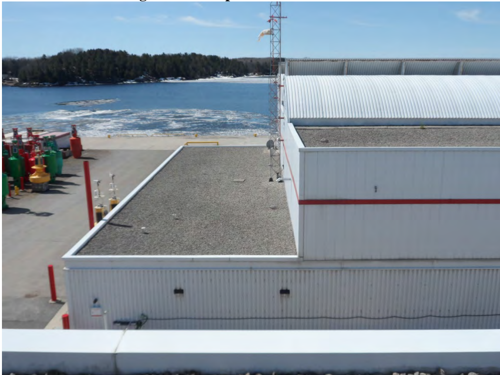
Photo 16: Helicopter Hanger ACM Sample HH-RF-03A,B,C and HH-RB-04A,B,C.
