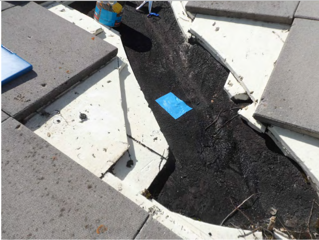
Photo 15: Main Bldg. ACM Sample MB-RF-02C.
