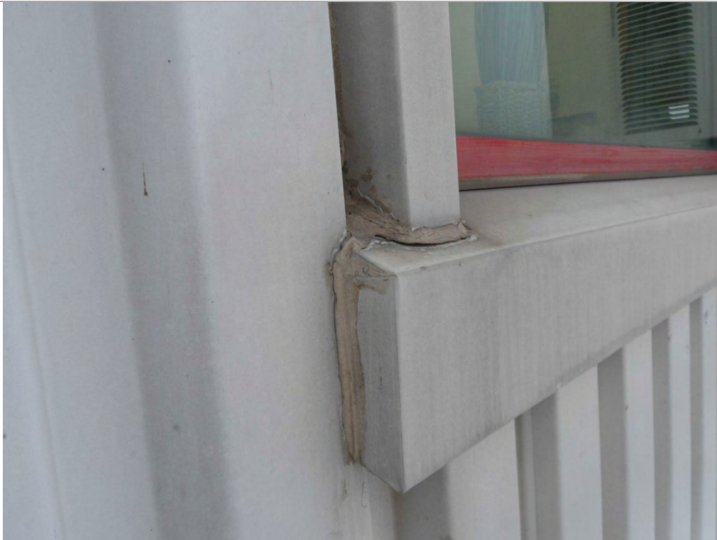
Photo 9: Main Building grey exterior siding paint - Lead-Containing (Sample Admin-P-30).
