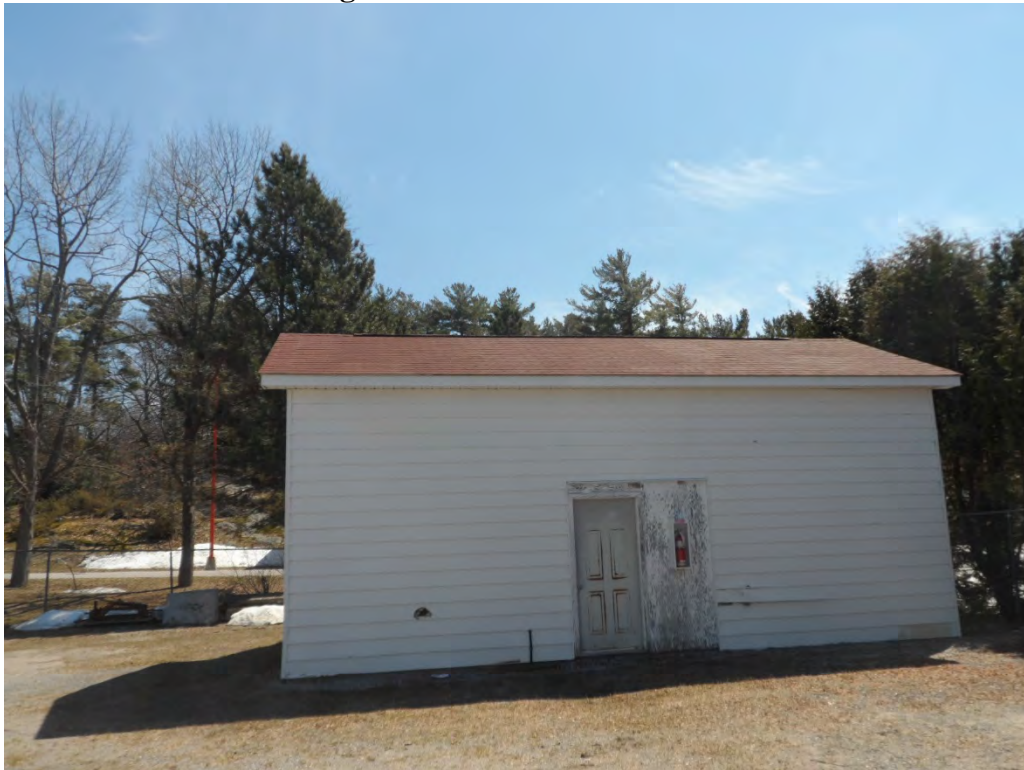
Photo 20: Garage (Samuel Risley Storage) recently replaced shingle roof.
