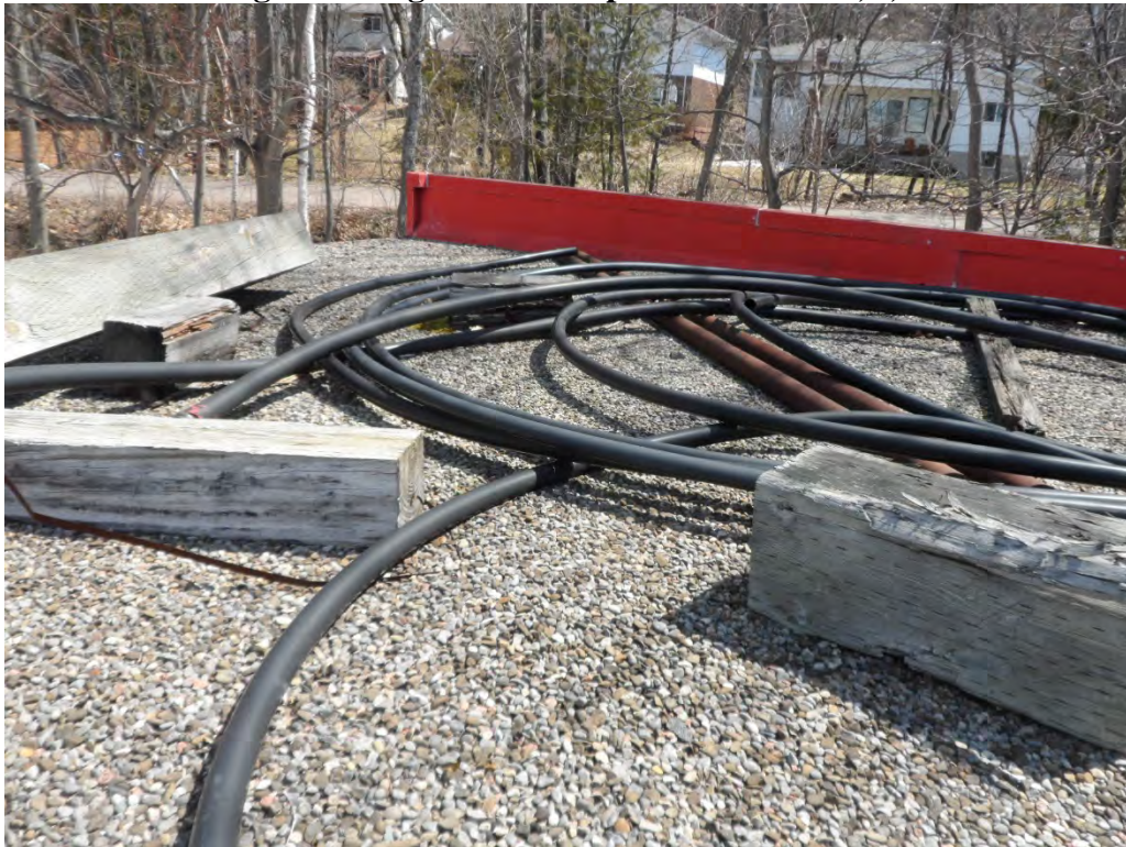
Photo 18: Winch House ACM Sample WH-RF-05A,B,C.
