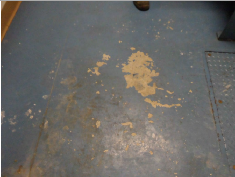
Photo 1: Main Building Room 179 blue interior floor paint – Lead-containing (Sample 179-P-12).
