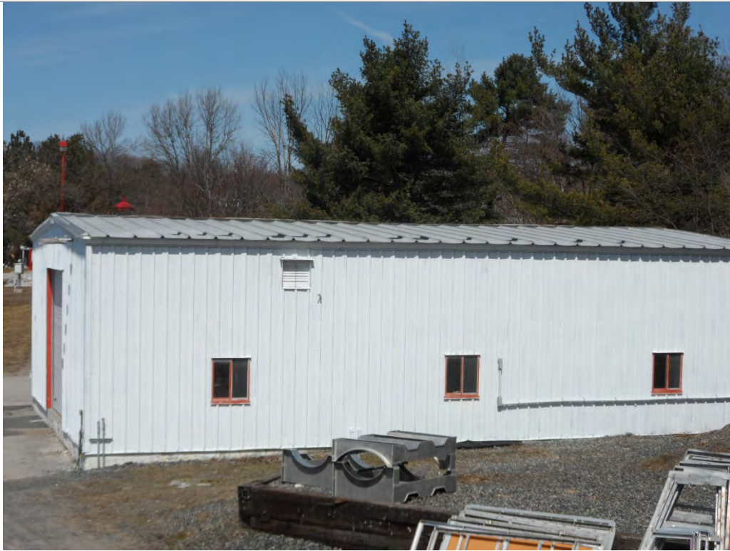
Photo 19: Marine Storage steel roof.
