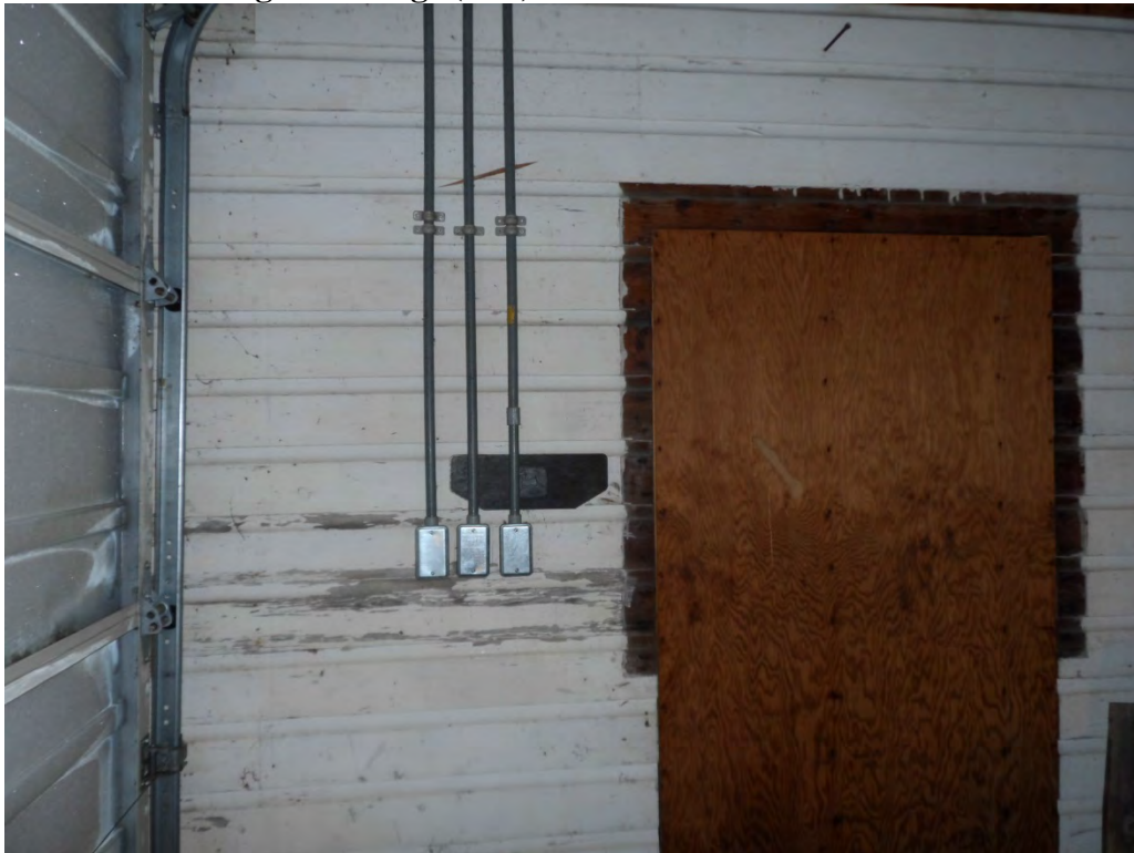
Photo 8: Storage Building (east) white interior siding paint – Lead-containing (Sample STR1-P-31).
