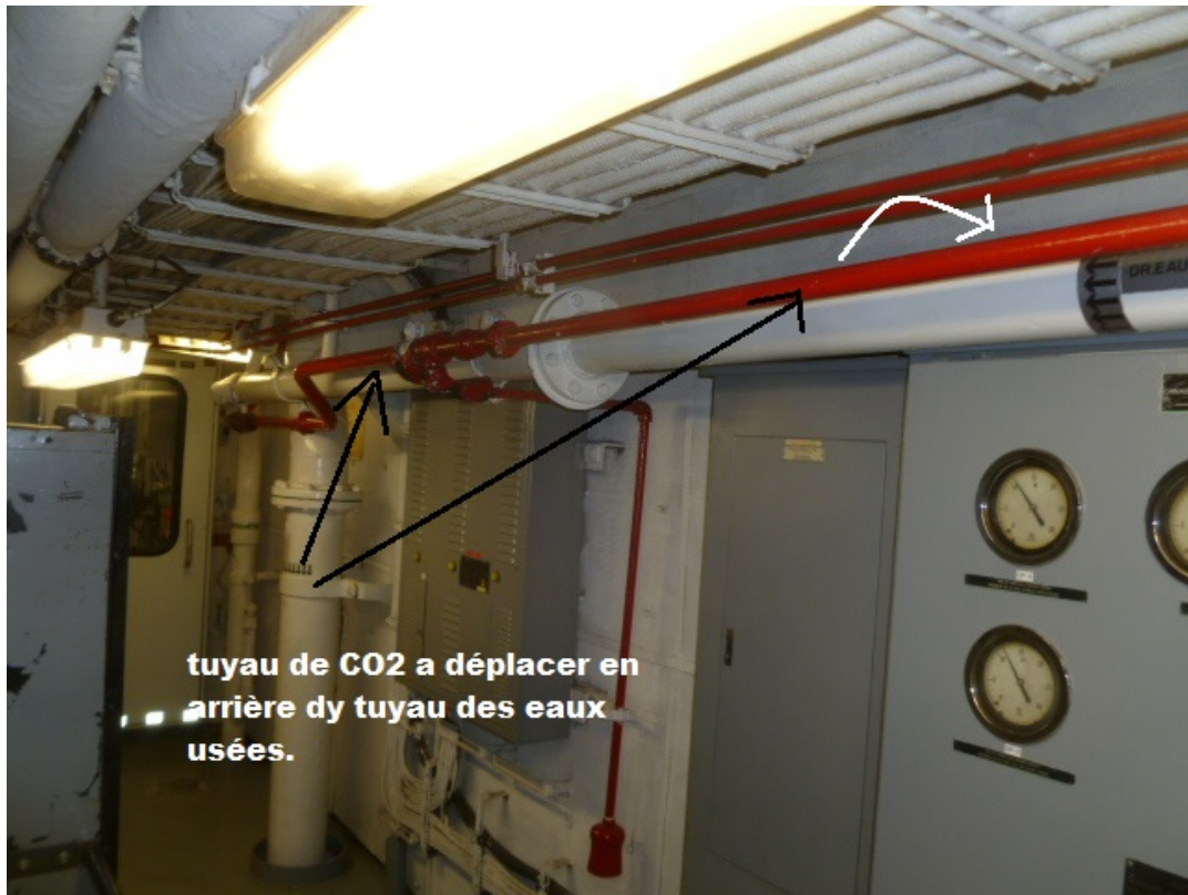
CO2 pipe to relocate on the outboard side of the adjacent grey water pipe
