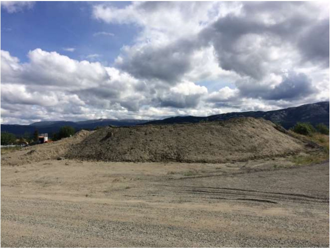
Photo 6: Compliant Stockpile in LTF to be used for backfill.
