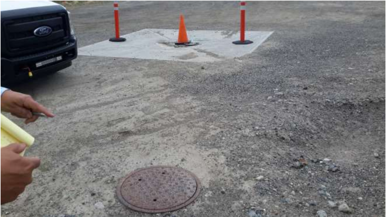
Photo 4: View of the manhole to the sanitary utility line and the sani dump in the background within the 'Optional Work' area.
