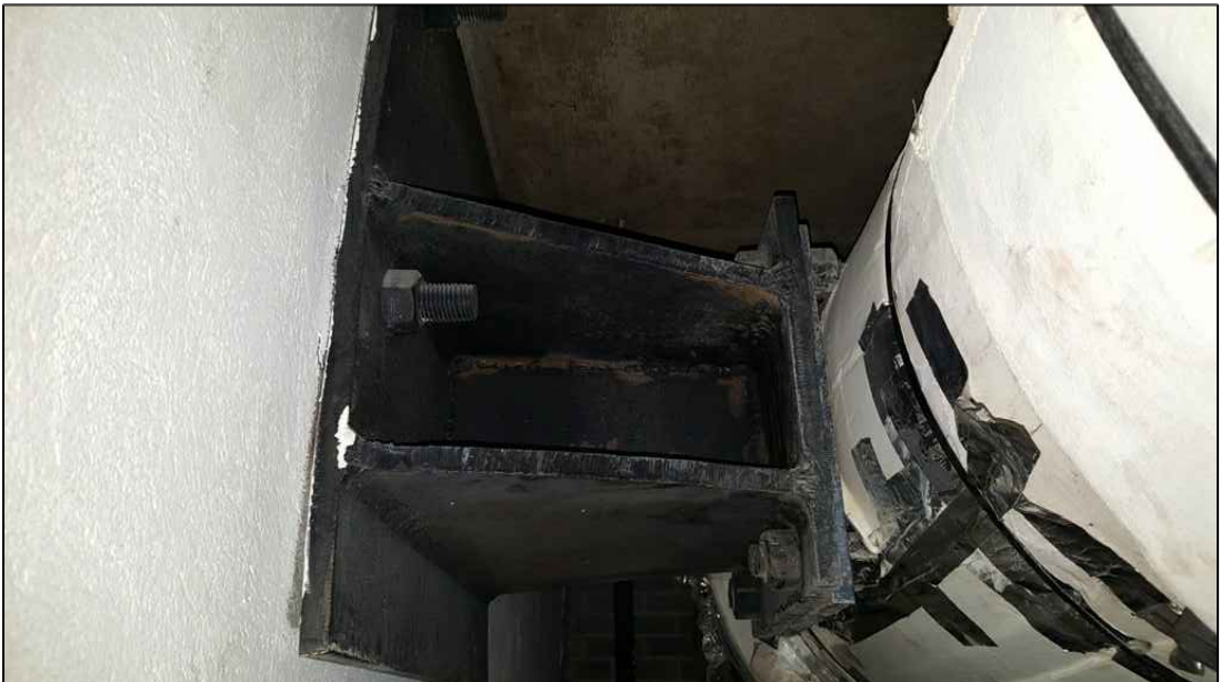
PHOTO 1—SIDE BRACKET BR-1 TO BE REPAIRED
