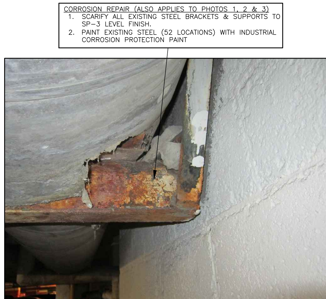
PHOTO 4—EXAMPLE OF CORROSION TO BE REPAIRED (52 REPAIR LOCATIONS REQ'D)
