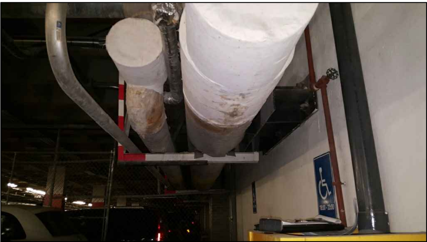
PHOTO 2—BEAM SIDE BRACKET BR-2 TO BE REPAIRED
