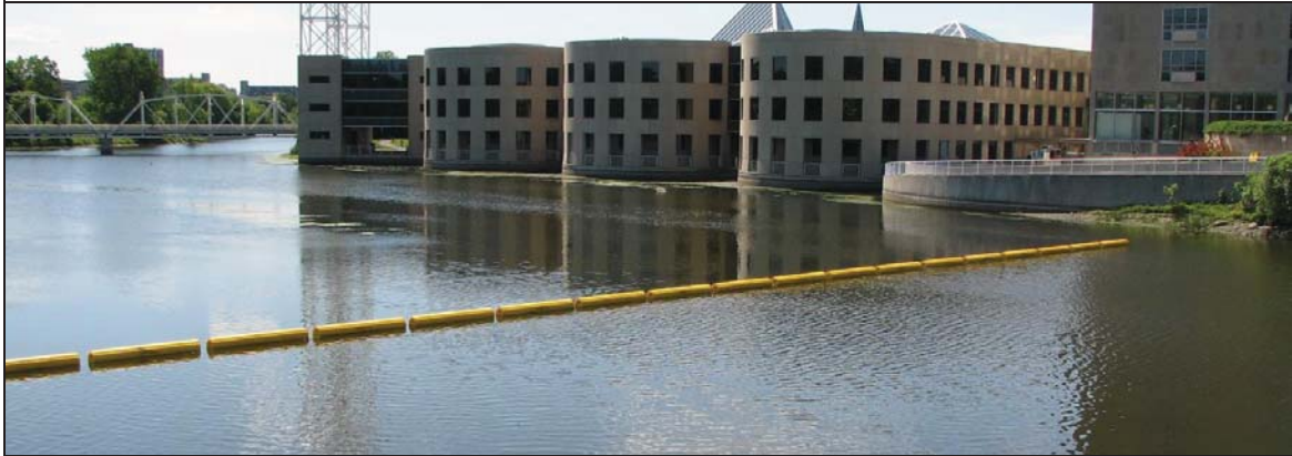
Figure 7 - Waterway barrier upstream of East Dam. A similar barrier is located upstream of the West Dam.
