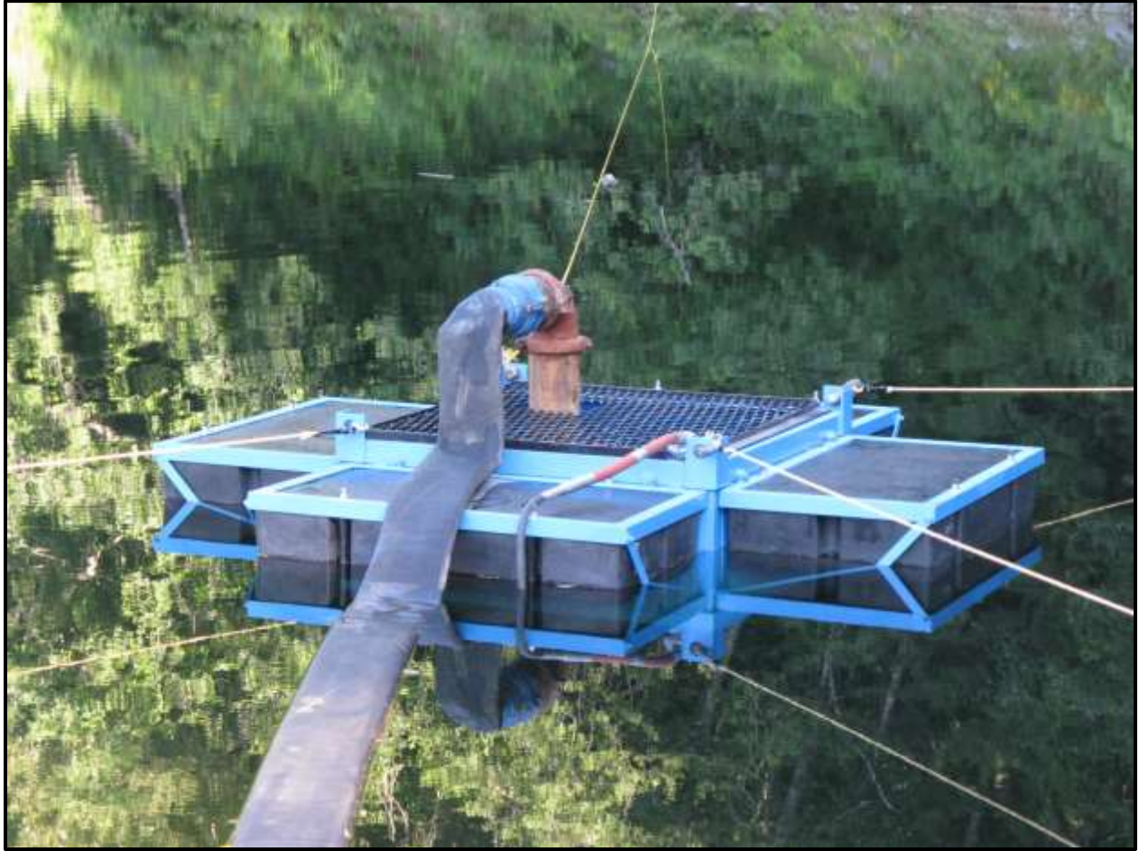
Figure 5: Floating cage used to house J205 submersible pumps. Three such pumps will be deployed in Johnson Lake in October 2017.
