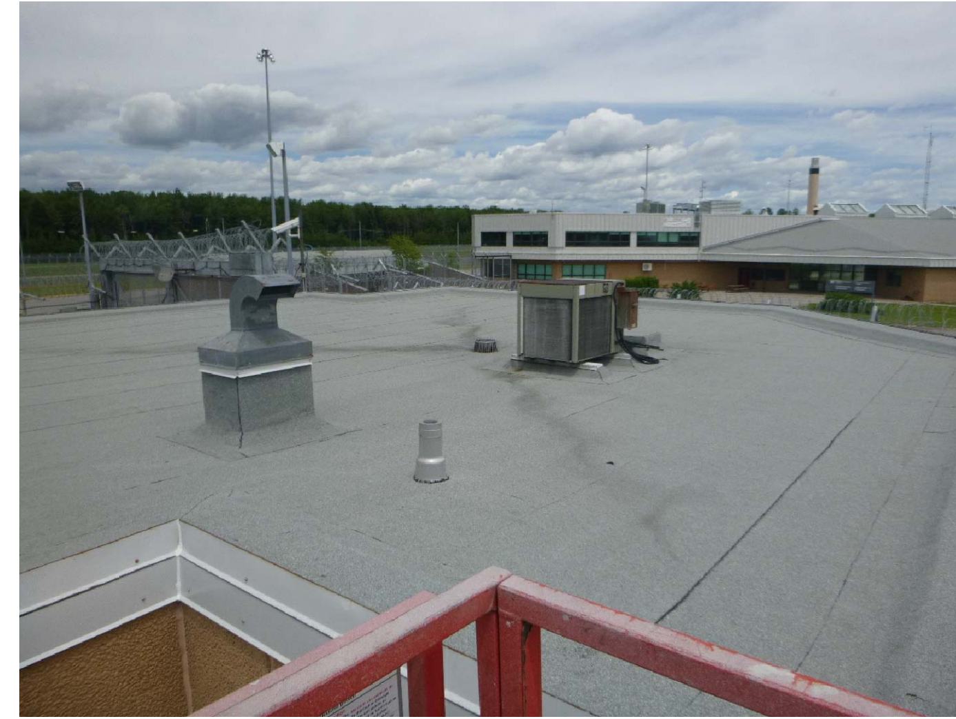
04 PICTURE - ROOF MECHANICAL SCALE: NONE
