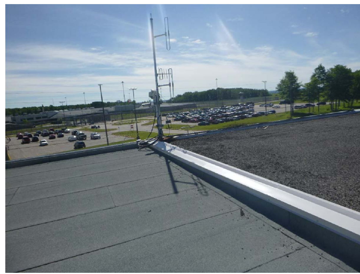
03 PICTURE - EXISTING ELECTRIC MAST SCALE: NONE
