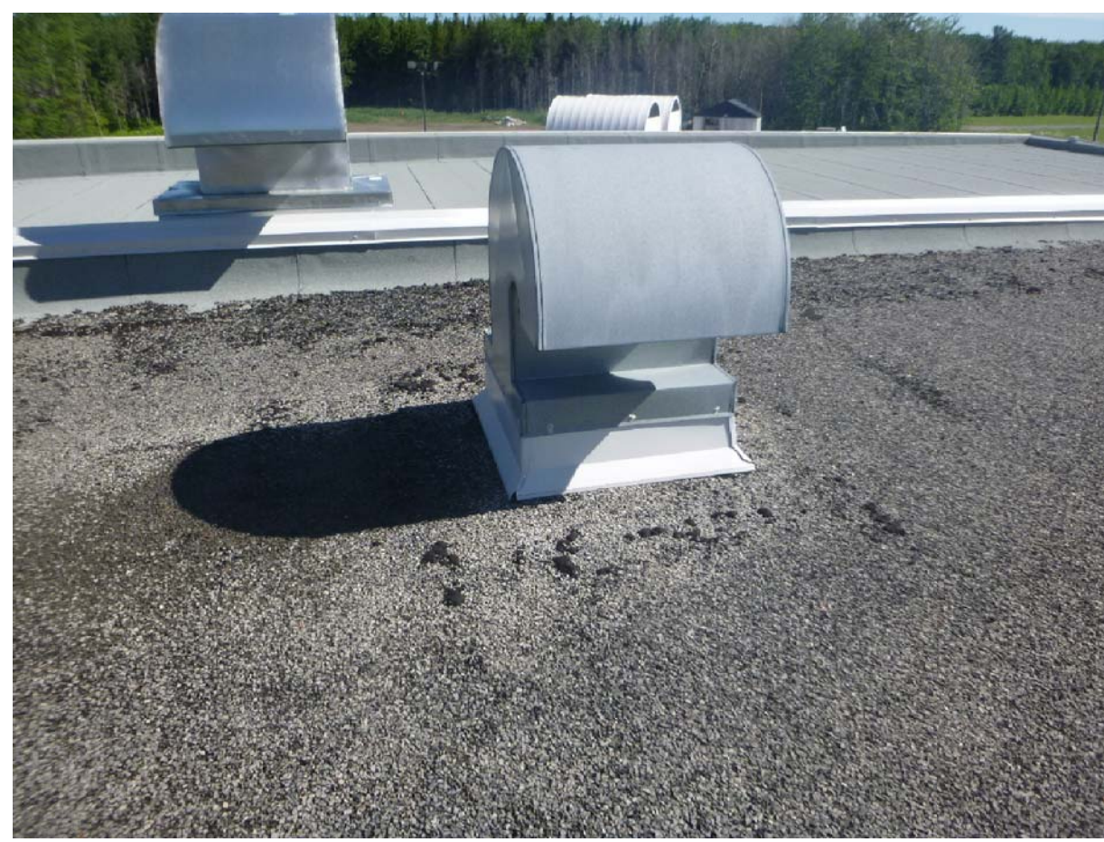
02 PICTURE - EXISTING GOOSENECK SCALE: NONE
