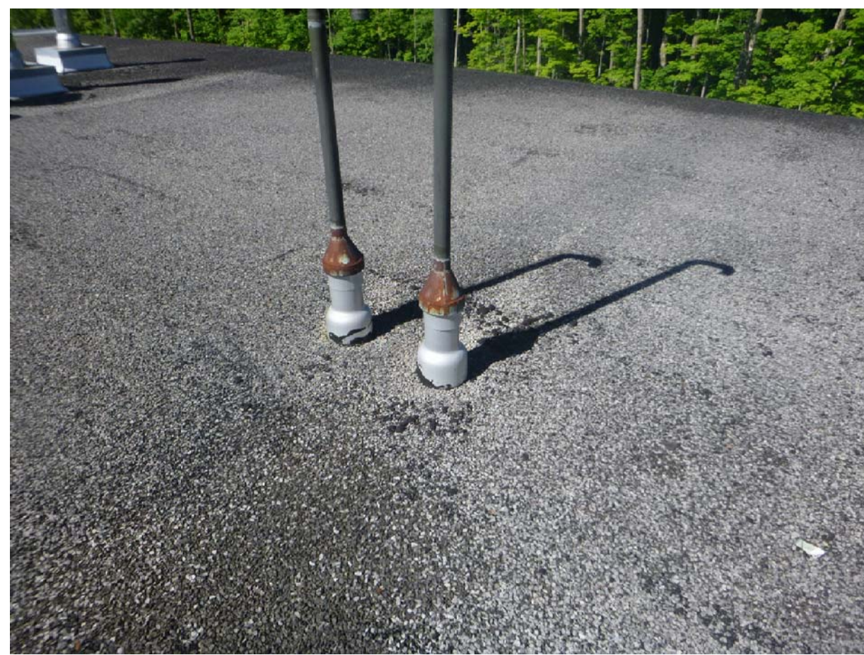
05 PICTURE - EXISTING CHIMNEY SCALE: NONE
