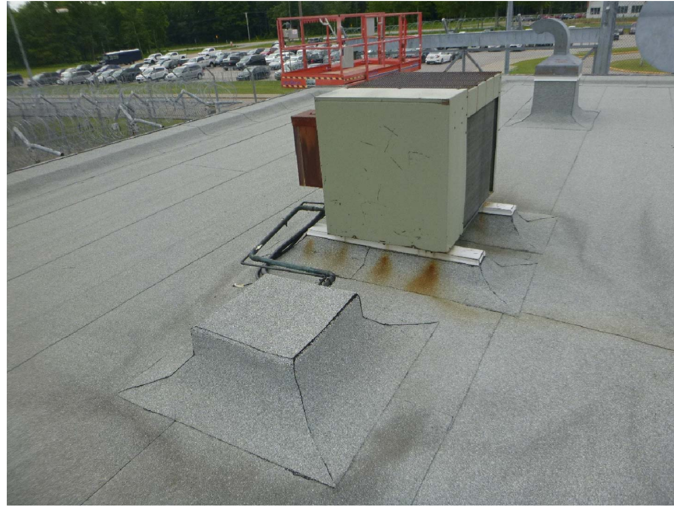
03 PICTURE - ROOF MECHANICAL SCALE: NONE
