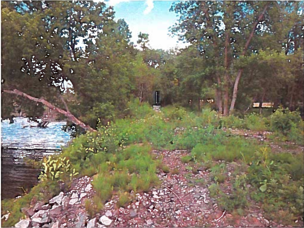
Photo 5. Earth dam on the north side of the overflow dam (May 2016).
