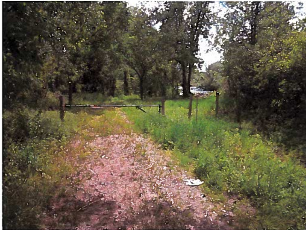
Photo 3. View of access road off of Hwy. 43. Likely access road and staging area for work on overflow dam and earth dam (May 2016).
