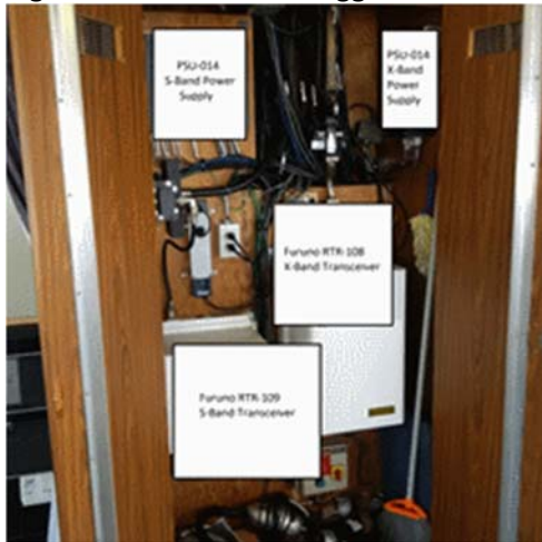
Figure 6: Radar Closet Suggested Furuno Radar locations
