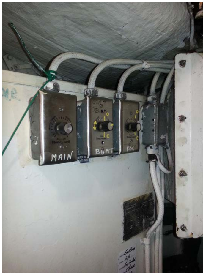
Figure 7. Control Dampers in Forecastle Machinery Space
