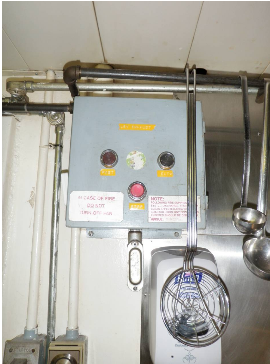
Figure 4. Galley ventilation controls (fast-slow-stop)
