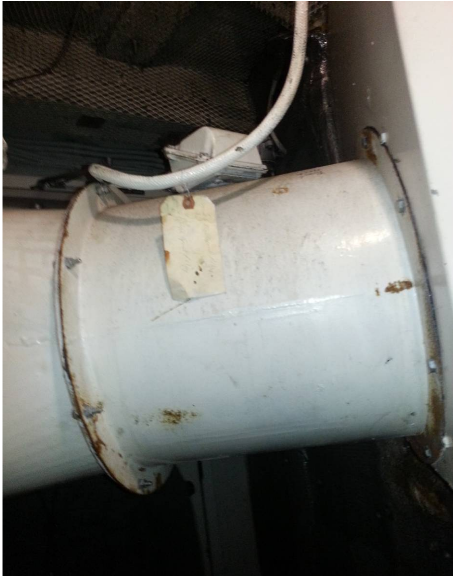
Figure 3. Fresh air fan ducted to louver
