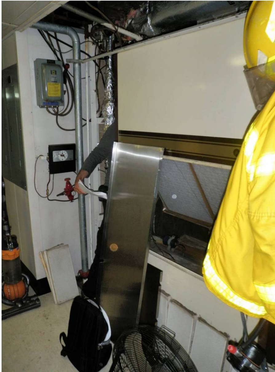
Figure 2. Main deck AC unit, with return air grille exposed
