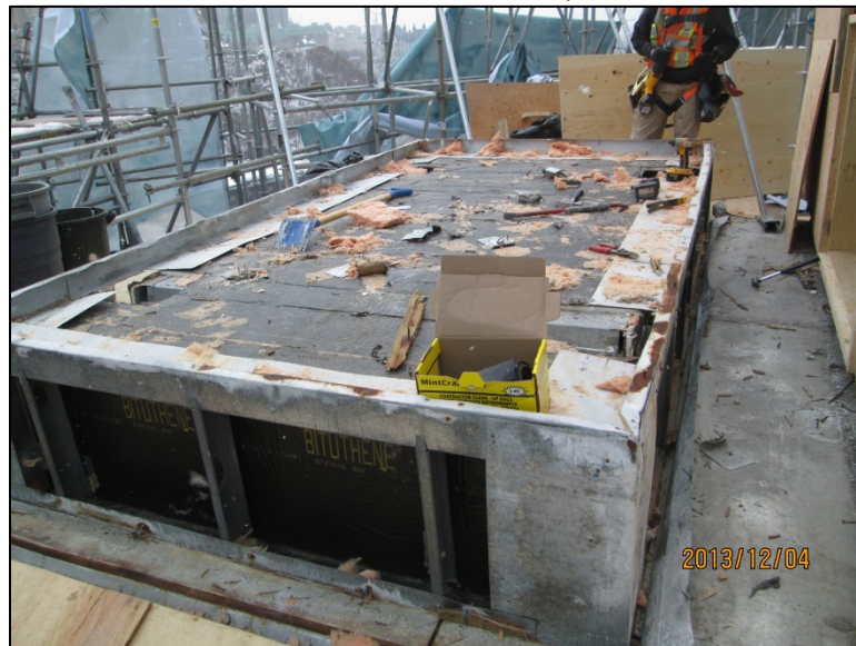
Similar roof – exterior elements removed
