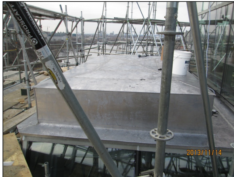
Similar roof – completed construction
