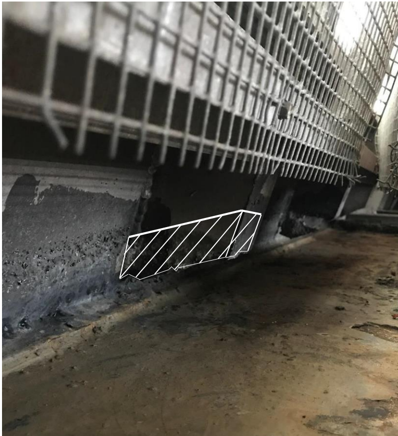
Photograph 1: Funnel side stiffeners to be cropped
