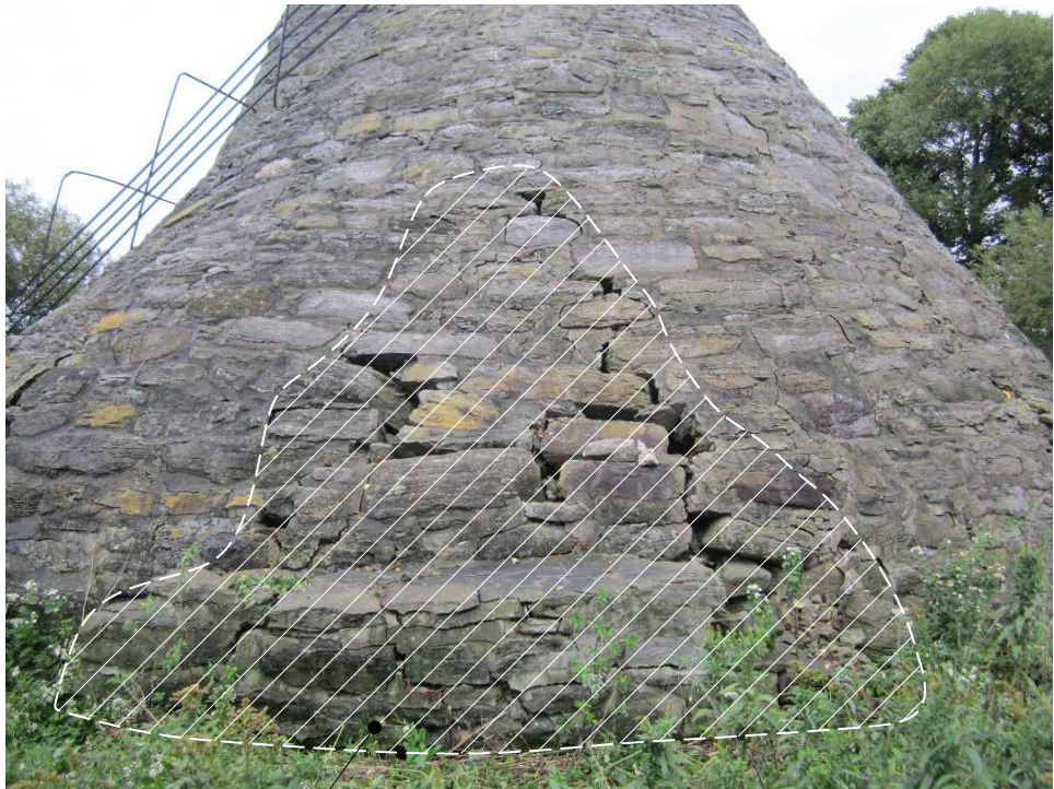
PHOTO 7 APPROXIMATE REPAIR AREA N.T.S.
