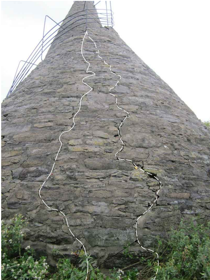
PHOTO 6 CRACK REPAIR AREA N.T.S.
