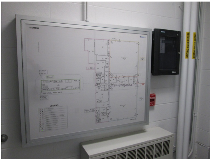
Fig. 54: Active Graphic and Remote Annunciator
