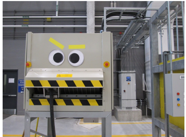
Fig. 52: 400Hz Aircraft Cable Reel
