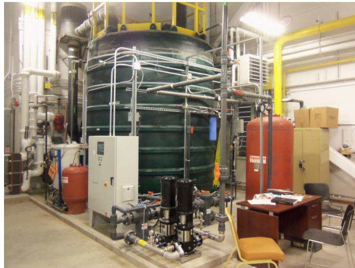
Fig. 10: Non Potable Water System
