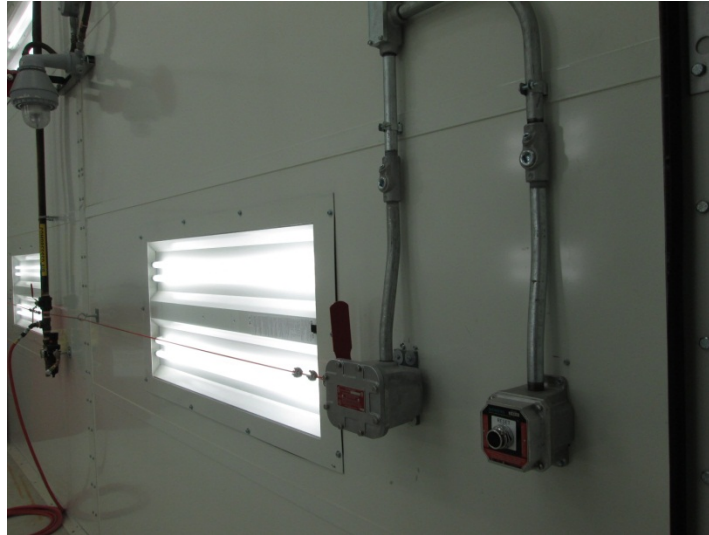
Fig. 56: Man Down Alarm Activation and Reset Units
