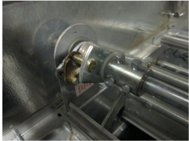
Fig. 17: Close-up of Fusible Link
