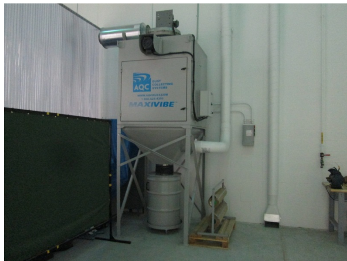
Fig. 29: Dust Collector
