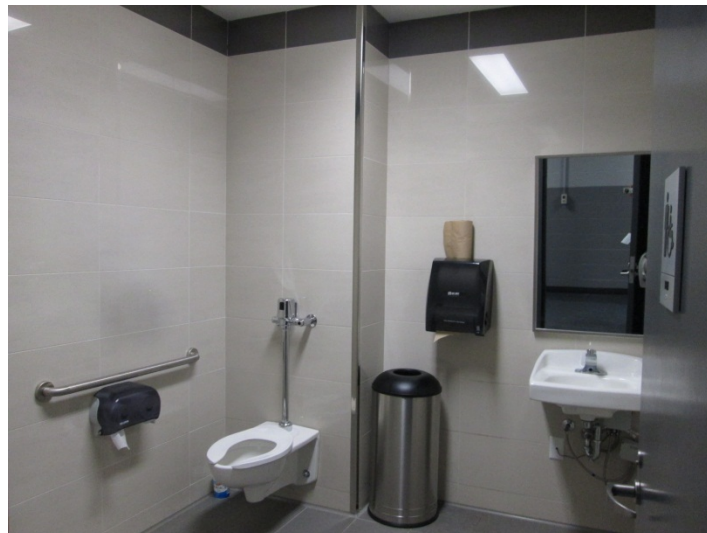
Fig. 11: Office Area Washroom
