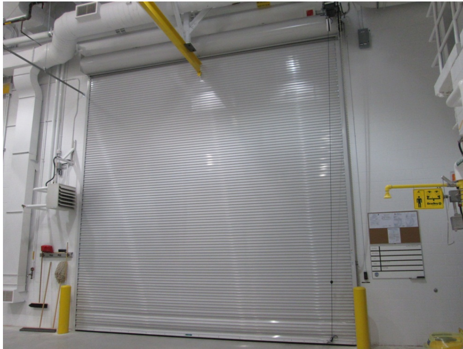
Fig. 1: Fire Rated Overhead Coiling Door
