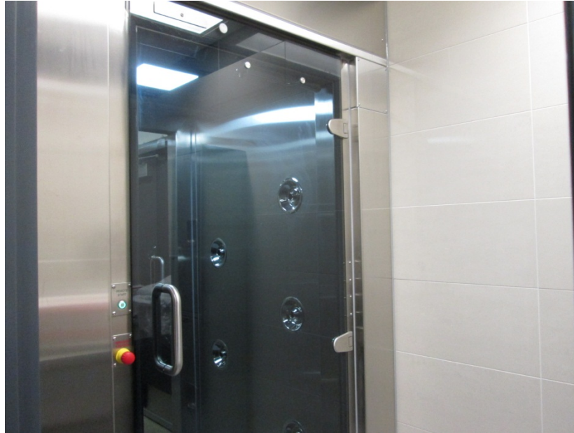
Fig. 6: Decontamination Shower
