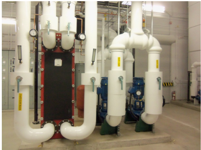
Fig. 24: Heat Exchanger # 1
