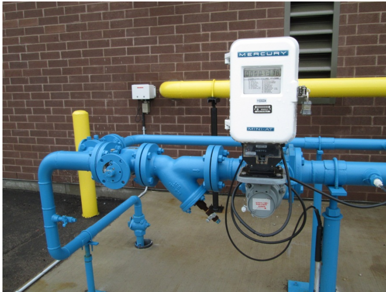
Fig. 36: Gas Meter
