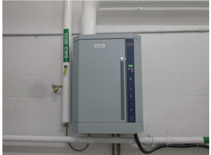
Fig. 34: Electric Humidifier, HUH7
