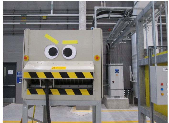
Fig. 52: 400Hz Aircraft Cable Reel
