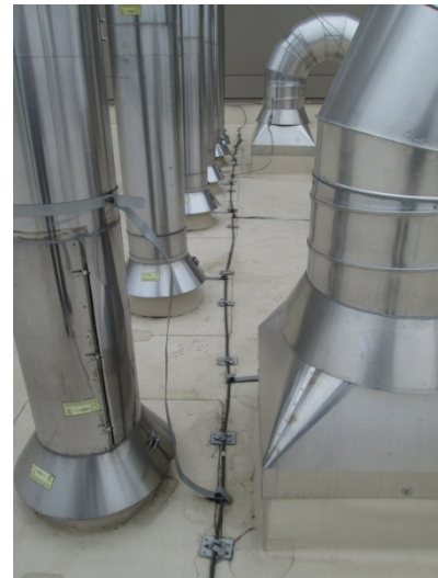
Fig. 48: Lightning Protection at Breaching
