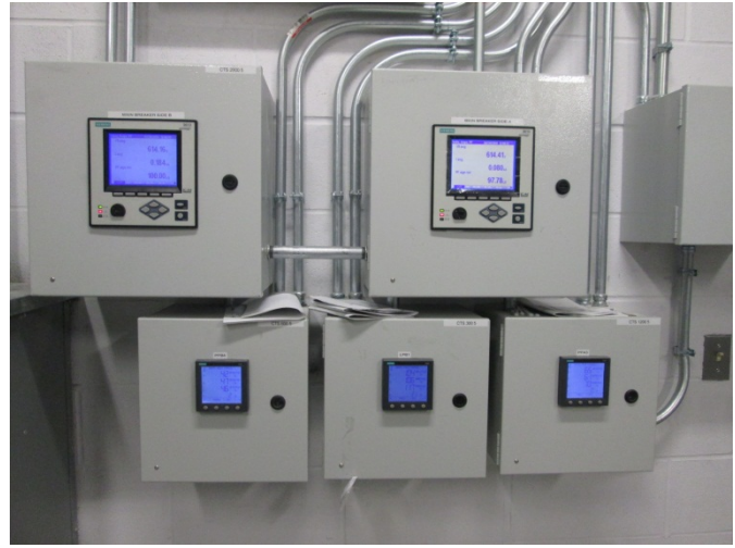
Fig. 41: Power Meters
