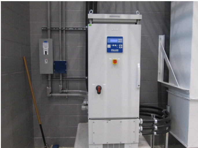
Fig. 51: 400Hz Frequency Converter
