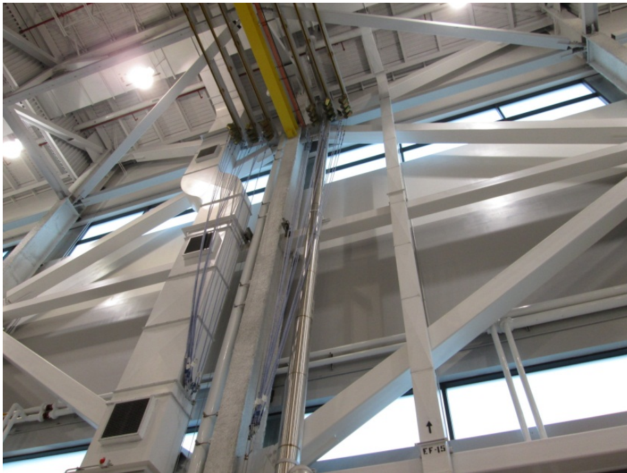
Fig. 5: Fall Arrest Tracks, Trolleys and Lifelines
