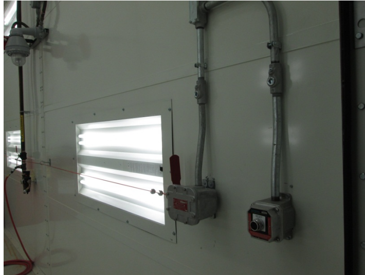
Fig. 56: Man Down Alarm Activation and Reset Units
