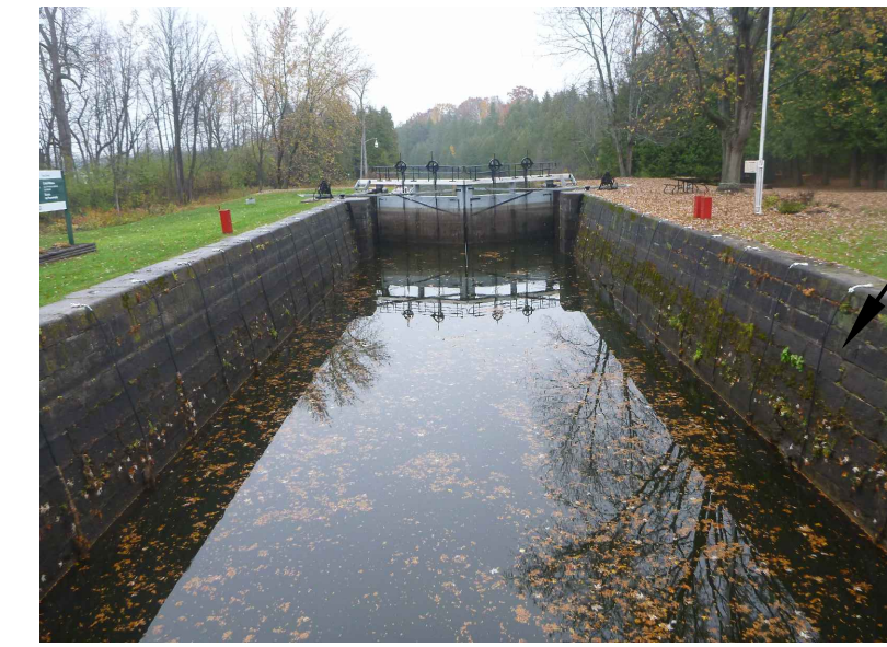
PHOTO 1 SCALE: NTS LOCK, LOOKING DOWNSTREAM 01 S06
