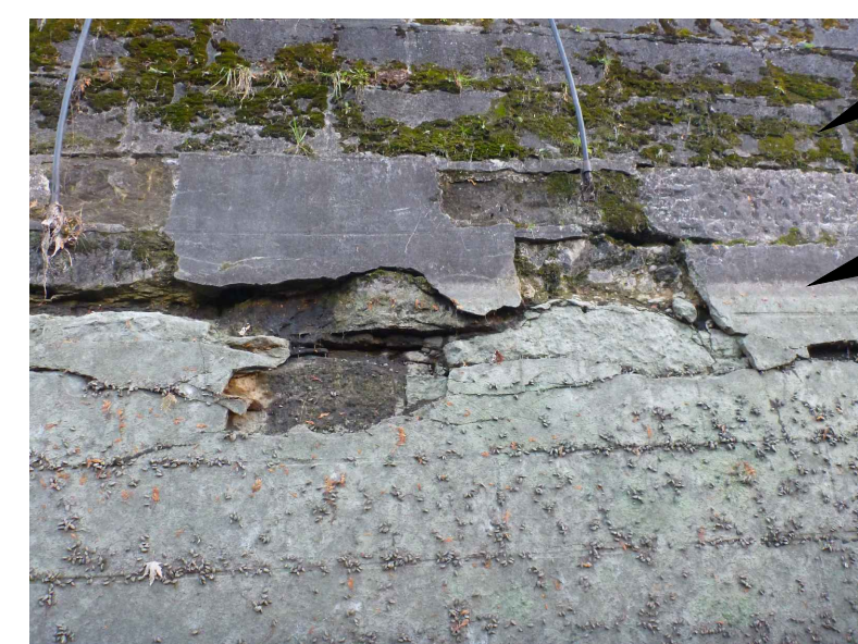
PHOTO 15 SCALE: NTS CLOSE UP SHOWING PARGING OVER STONE FACE 15 S06
