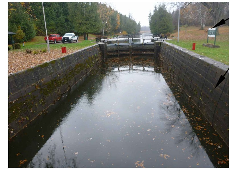
PHOTO 2 SCALE: NTS LOCK, LOOKING UPSTREAM 02 S06
