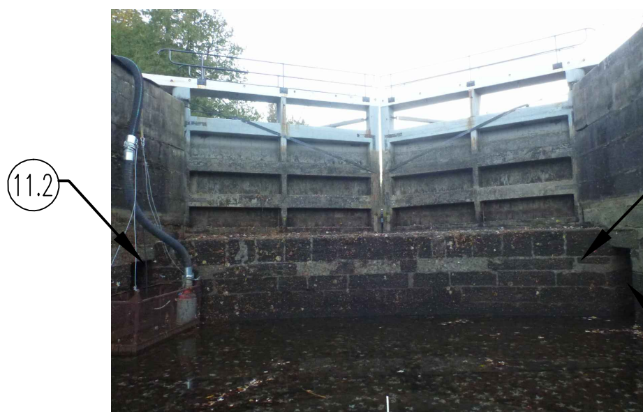
PHOTO 11 SCALE: NTS UPSTREAM BREAST WALL 11 S06
