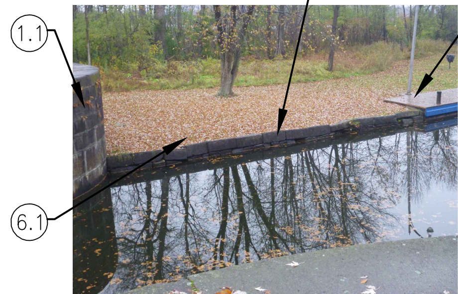
PHOTO 6 SCALE: NTS DOWNSTREAM WEST APPROACH WALL 06 S06
