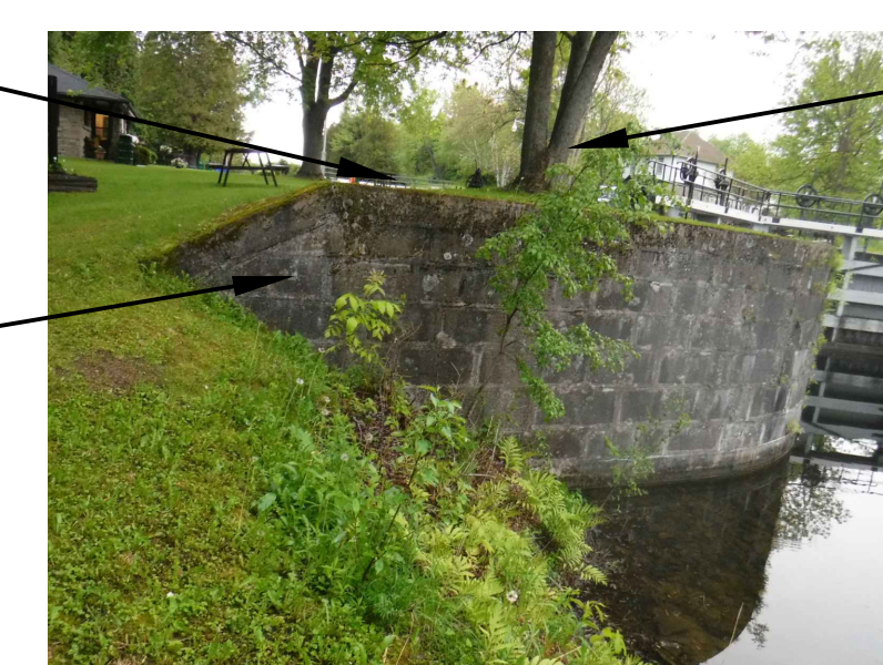
PHOTO 22 SCALE:NTS NORTH EAST WING WALL
