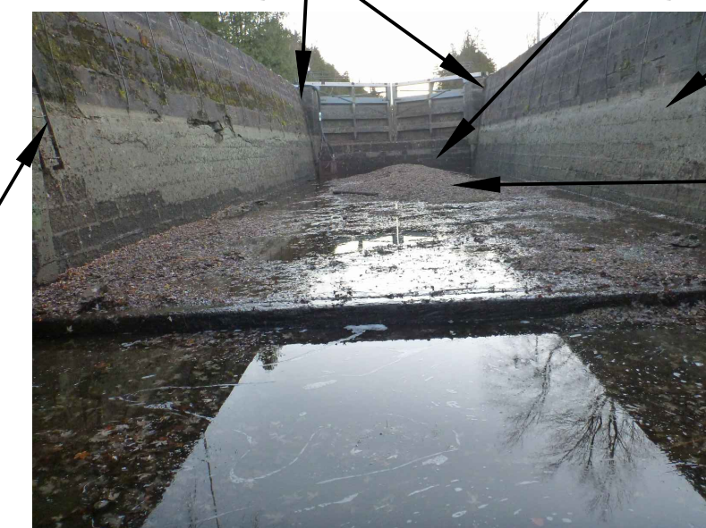
PHOTO 12 SCALE: NTS LOCK FLOOR (LOOKING UPSTREAM) 12 S06
