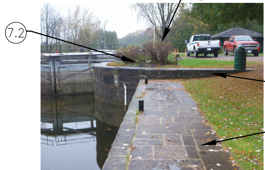
PHOTO 7 SCALE: NTS UPSTREAM EAST APPROACH WALL AND WING WALL 07 S06
