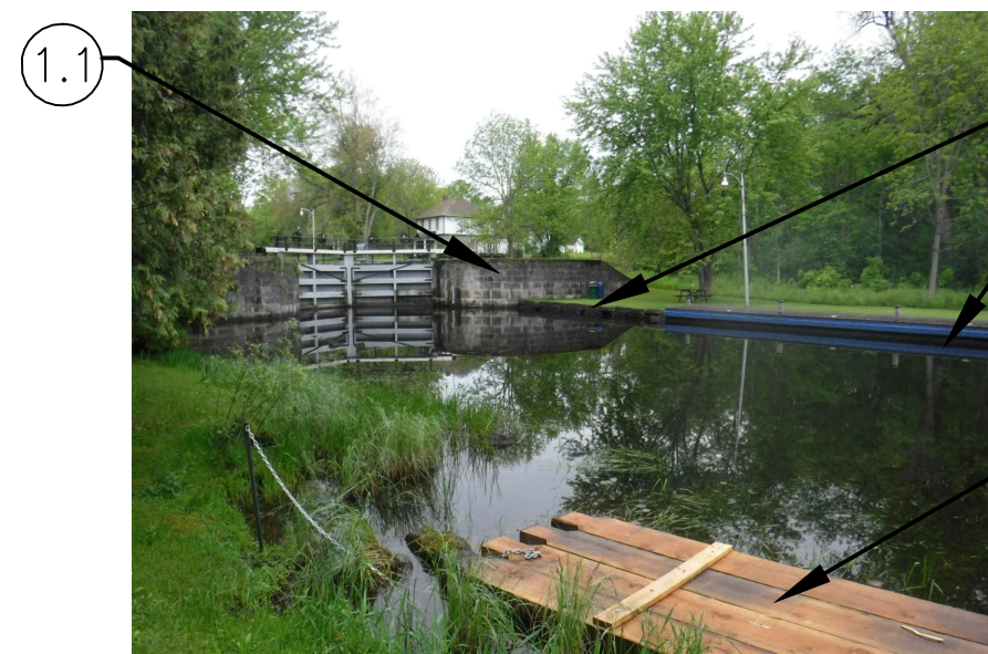
PHOTO 5 SCALE: NTS DOWNSTREAM WING WALLS 05 S06
