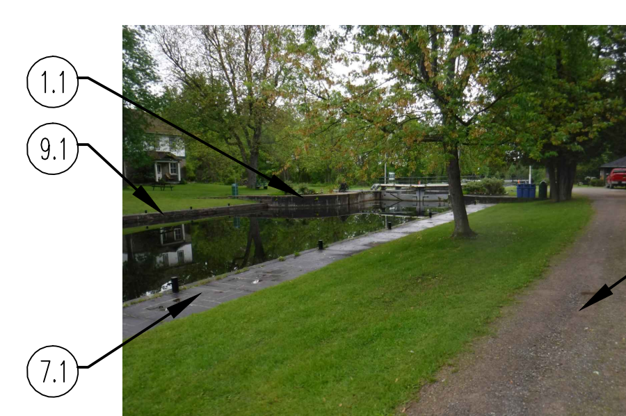
PHOTO 28 SCALE:NTS LOCK SITE LOOKING NORTH
