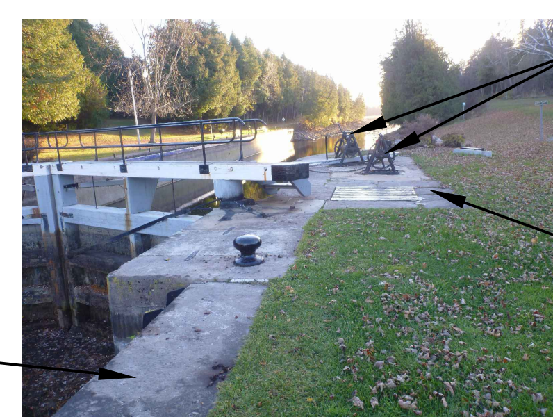
PHOTO 21 SCALE:NTS SKYWARD FACING MASONRY AND CONCRETE
