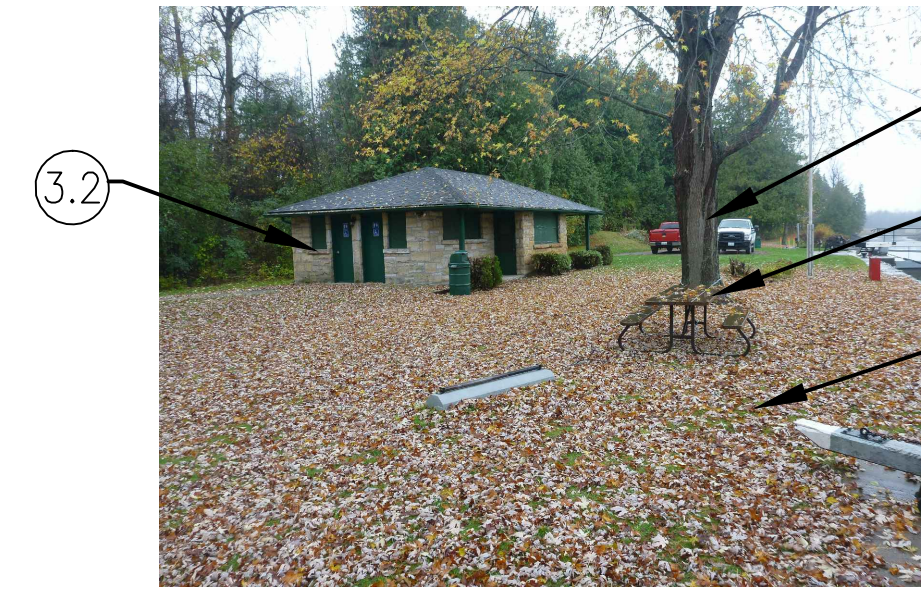
PHOTO 3 SCALE: NTS PCA LOCKSTATION OFFICE/POSSIBLE STAGING AREA 03 S06
