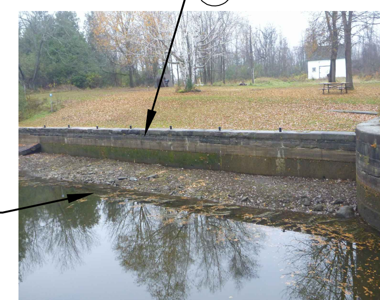
PHOTO 32 SCALE:NTS DOWNSTREAM WEST APPROACH WALL
