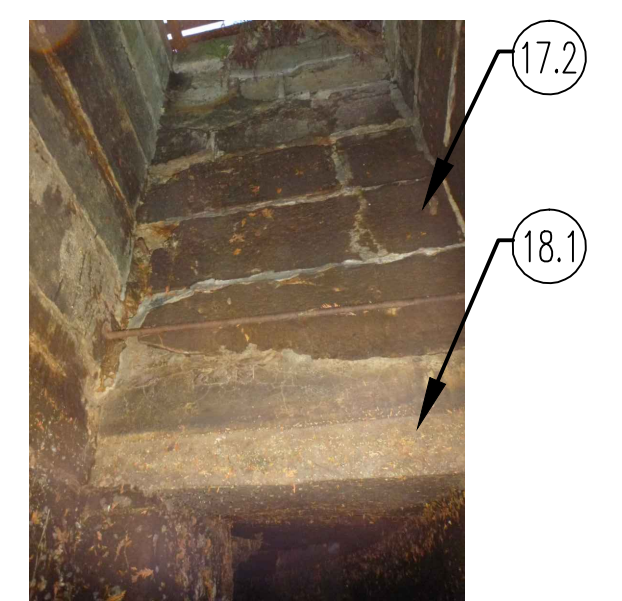
PHOTO 19 SCALE:NTS WEST SLUICE VENT AND TUNNEL
