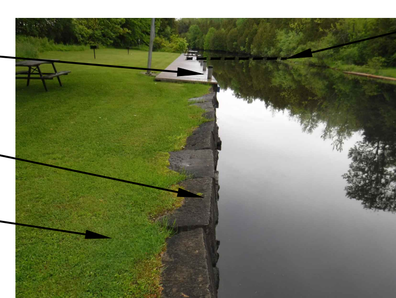
PHOTO 25 SCALE:NTS DOWNSTREAM WEST APPROACH WALL
