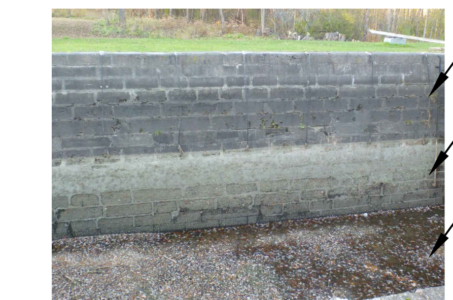
PHOTO 13 SCALE: NTS WEST LOCK WALL 13 S06
