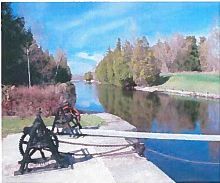
Figure 8 - Upstream view from lock
