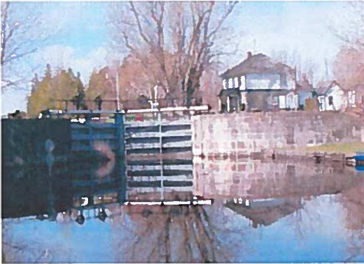
Figure 7 - Lockmaster's House and Lock
