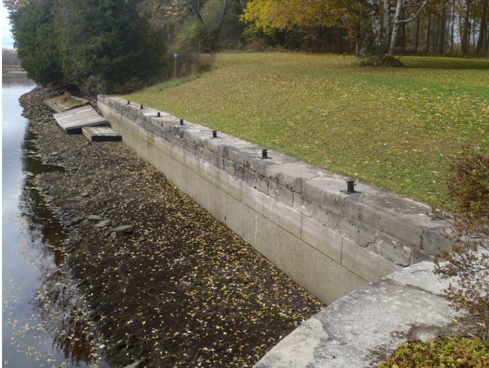
Photo 1. Dewatered cut immediately upstream of Poonamalie Lockstation (May 2016).
