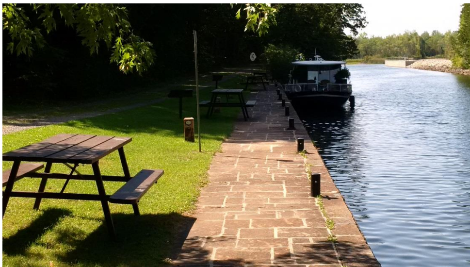
Photo 3. View looking upstream from the Poonamalie lockstation towards the earth dam.
