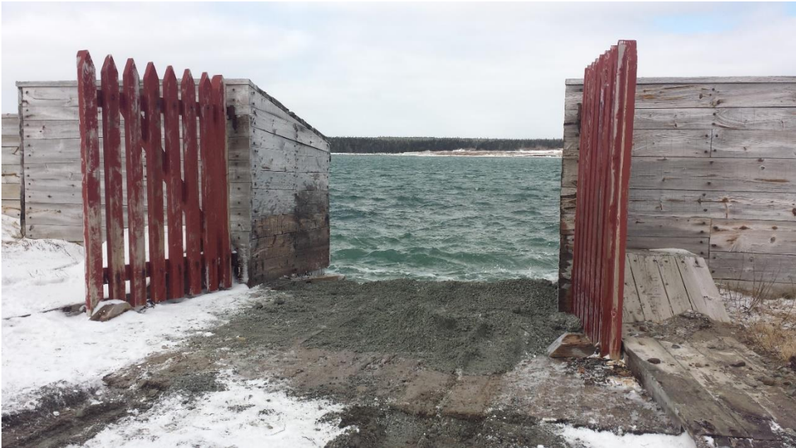
Photo 3. Quay Wall Cale (Gemtec, March 2017).
