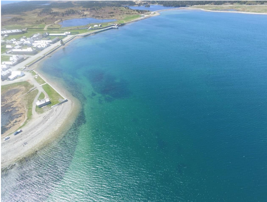
Photo 5. View of Quay Wall (note deposited sediment) (DFO, June 2017).
