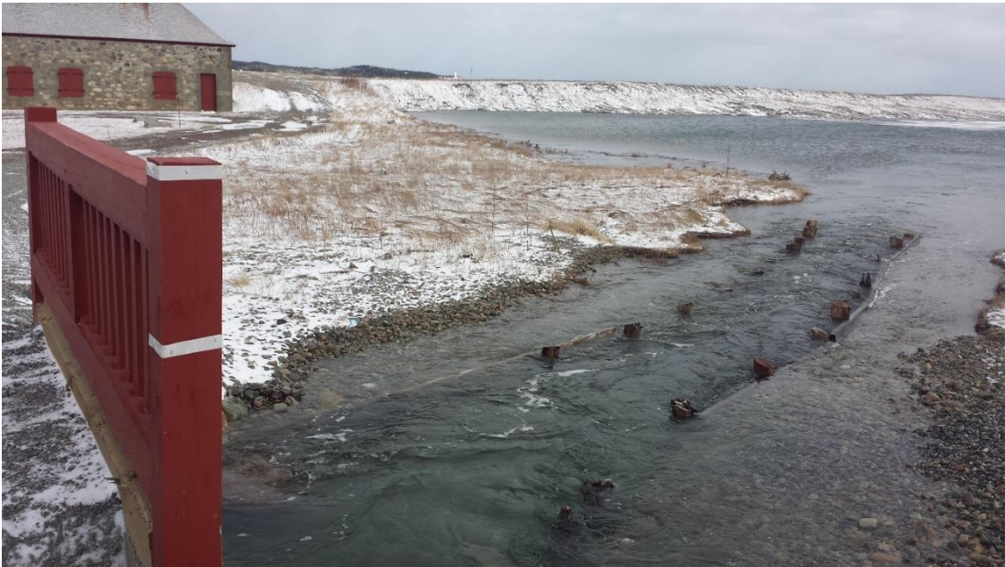
Photo 9. Grand Étang Pond draining through entrance of sluiceway (Gemtec, March 2017).
