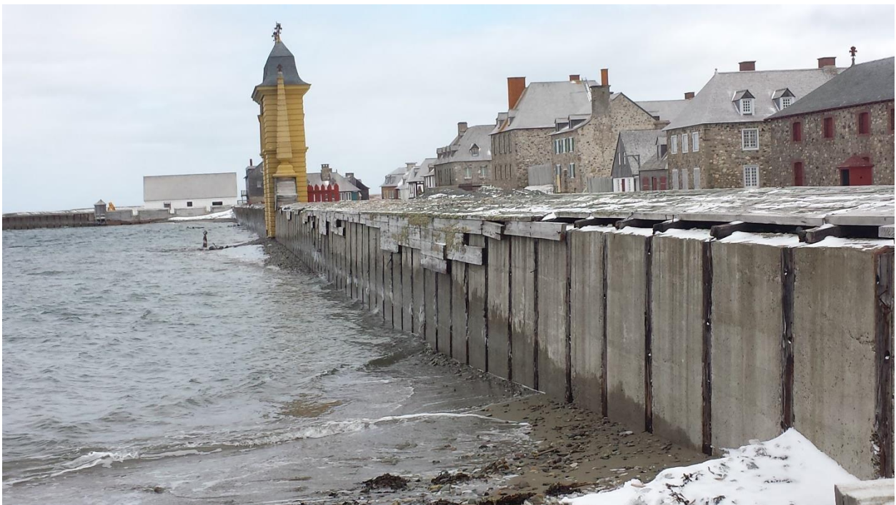
Photo 4. Sediment deposited along the Quay Wall (Gemtec, March 2017).
