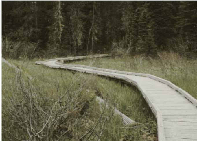
Figure 4.1 Wood treated with waterborne preservatives is often used for decking, such as in this wetland boardwalk (Lebow and Tippie, 2001).
