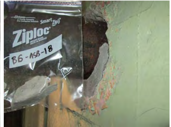
Photo 21: View of concrete block mortar sample BS-ASB-18.
