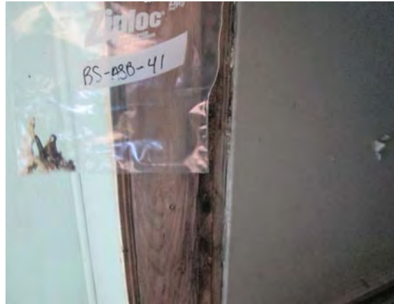
Photo 44: View of beige caulking sample BS-ASB-41.
