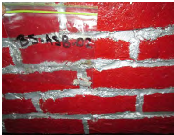
Photo 5: View of brick mortar sample BS-ASB-02.
