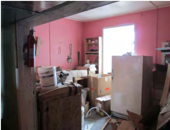
Photo 172: View of refrigerator in duplex dwelling storage room 1.
