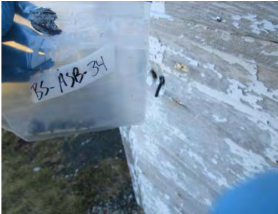
Photo 37: View of black caulking sample BS-ASB-34.
