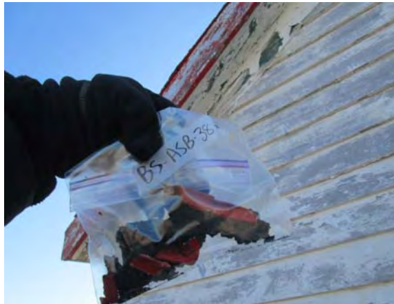
Photo 41: View of black asphalt shingle sample BS-ASB-38.
