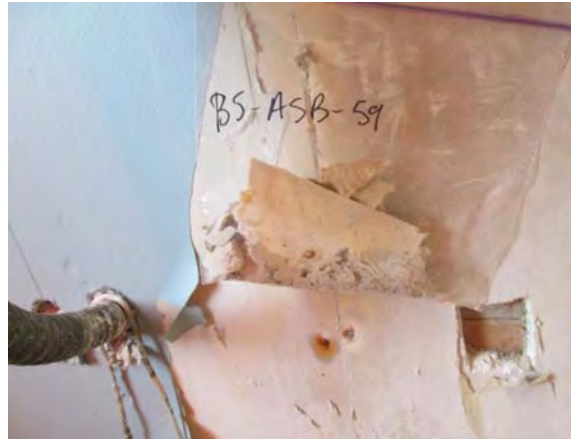
Photo 62: View of drywall joint compound sample BS-ASB-59.
