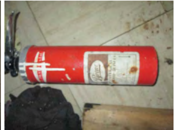
Photo 177: View of fire extinguisher in duplex dwelling pantry.
