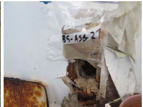
Photo 30: View of fibreglass insulation sample BS-ASB-27.
