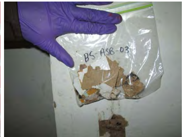
Photo 6: View of drywall joint compound sample BS-ASB-03.
