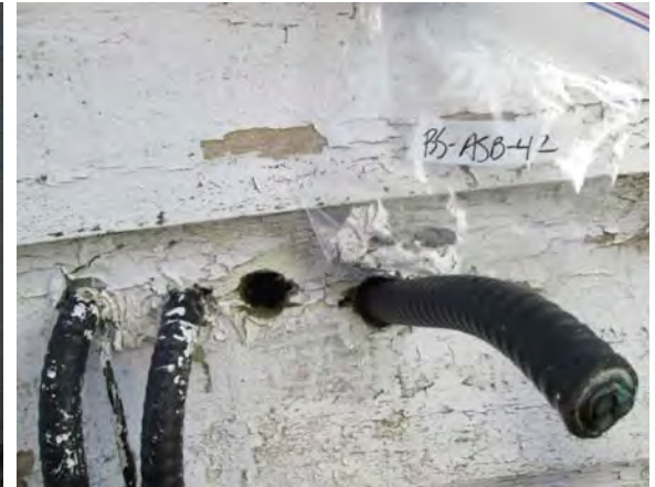
Photo 45: View of grey caulking sample BS-ASB-42.
