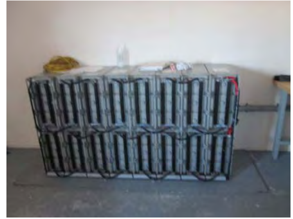
Photo 183: View of solar batteries in videograph building.
