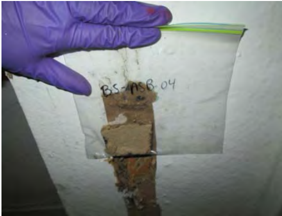
Photo 7: View of wood fibreboard sample BS-ASB-04.
