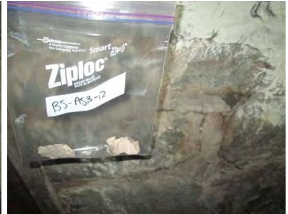
Photo 15: View of concrete block mortar sample BS-ASB-12.
