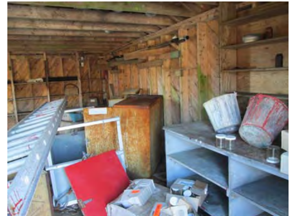
Photo 174: View of freezer in storage shed 1.
