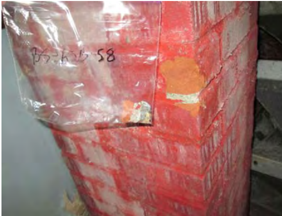
Photo 61: View of grey brick mortar sample BS-ASB-58.
