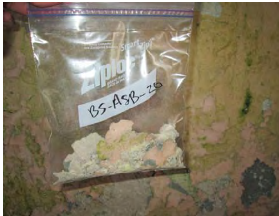
Photo 23: View of concrete parging sample BS-ASB-20.
