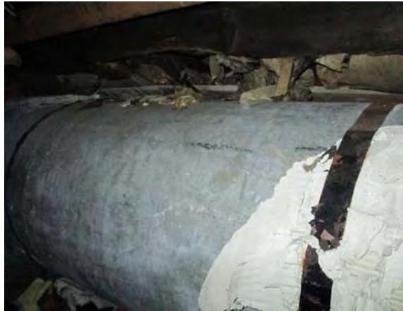
Photo 20: View of location of cardboard-type insulation sample BS-ASB-17.
