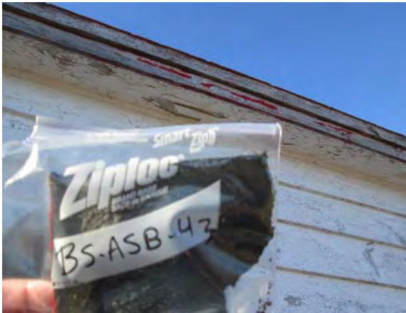
Photo 46: View of black asphalt shingle with tar paper sample BS-ASB-43.
