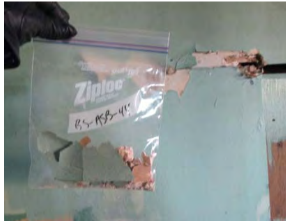
Photo 47: View of drywall joint compound and plaster sample BS-ASB-44.
