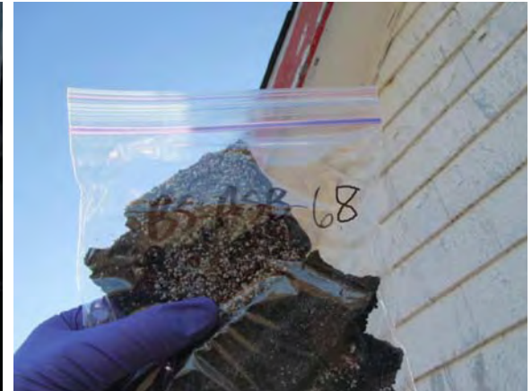
Photo 57: View of asphalt shingle sample BS-ASB-54. Note: sample ID revised.
