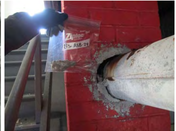
Photo 27: View of brick mortar sample BS-ASB-24.
