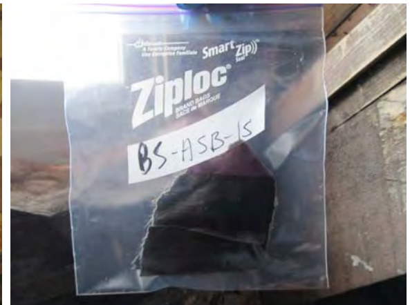
Photo 18: View of fibreglass insulation with paper backing sample BS-ASB-15.
