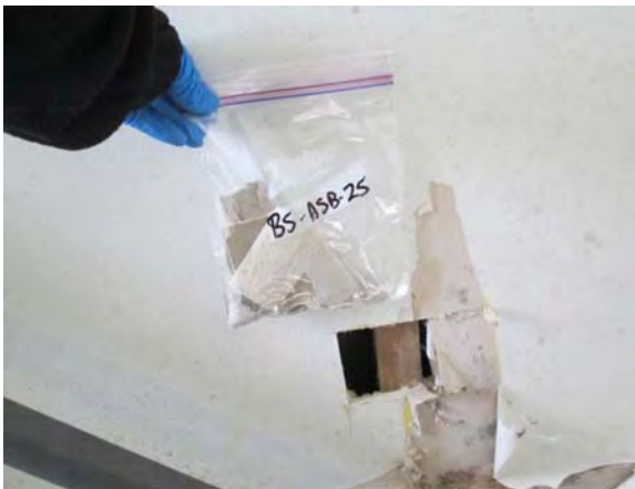
Photo 28: View of drywall joint compound sample BS-ASB-25.
