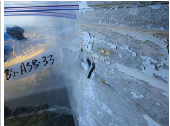
Photo 36: View of grey caulking sample BS-ASB-33.
