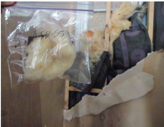
Photo 58: View of fibreglass insulation sample BS-ASB-55.
