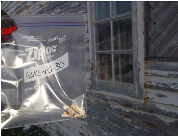
Photo 34: View of window caulking sample GULL-AS-30.
