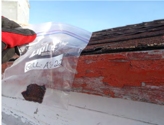
Photo 26: View of asphalt shingle sample GULL-AS-22.
