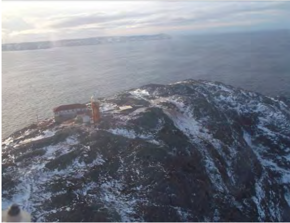
Photo 1: View of the Upper Landing Area, Gull Island Lightstation, NL.
