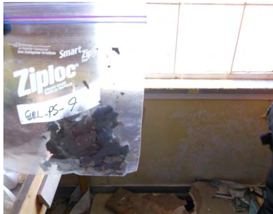
Photo 53: View of paint sample GULL-PS-9.
