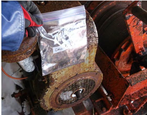
Photo 80: View of paint sample GULL-PS-36.
