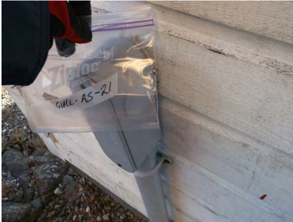
Photo 25: View of electrical conduit caulking sample GULL-AS-21.
