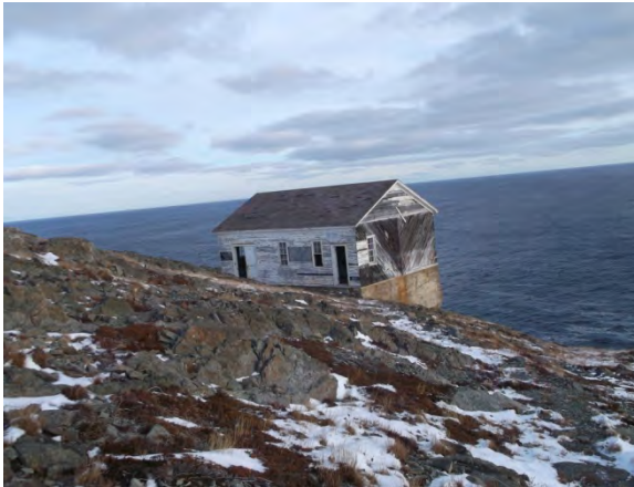
Photo 4: View of the Lower Equipment Building Area, Gull Island Lightstation, NL.
