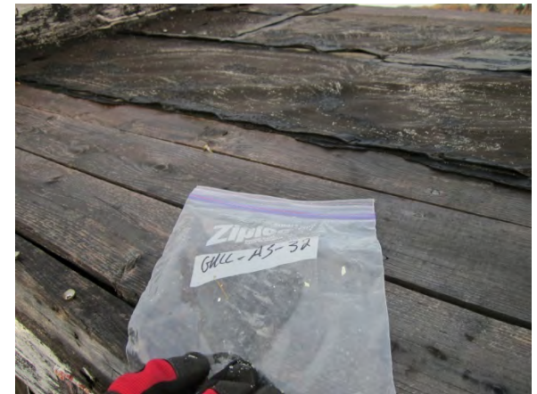
Photo 36: View of asphalt shingle sample GULL-AS-32.
