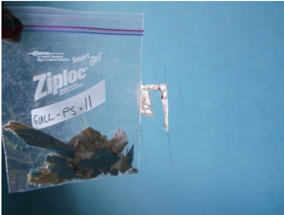
Photo 55: View of paint sample GULL-PS-11.
