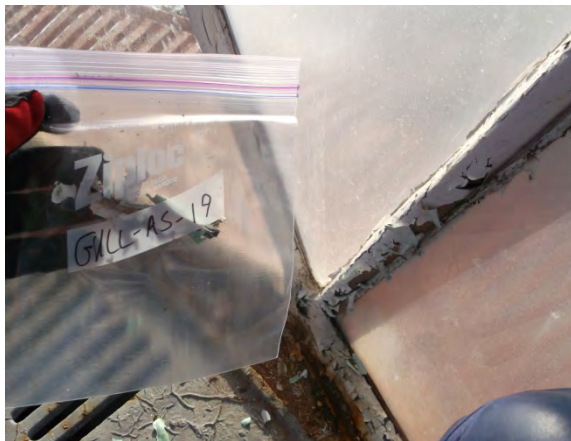
Photo 23: View of window caulking sample GULL-AS-19.
