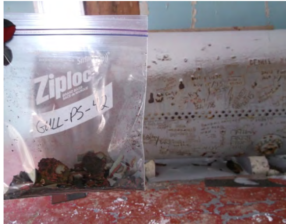
Photo 86: View of paint sample GULL-PS-42.
