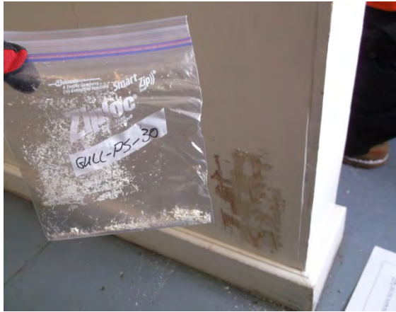
Photo 74: View of paint sample GULL-PS-30.
