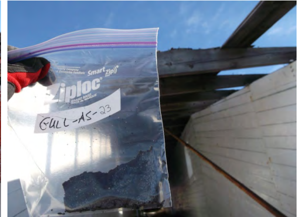
Photo 27: View of asphalt Shingle sample GULL-AS-23.
