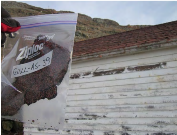
Photo 43: View of asphalt shingle sample GULL-AS-39.
