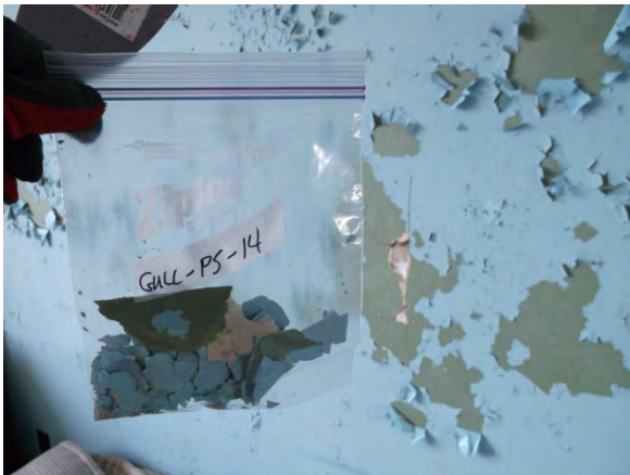
Photo 58: View of paint sample GULL-PS-14.
