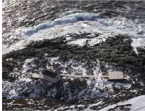
Photo 2: View of the Lower Landing Area, Gull Island Lightstation, NL.
