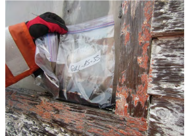
Photo 39: View of window caulking sample GULL-AS-35.
