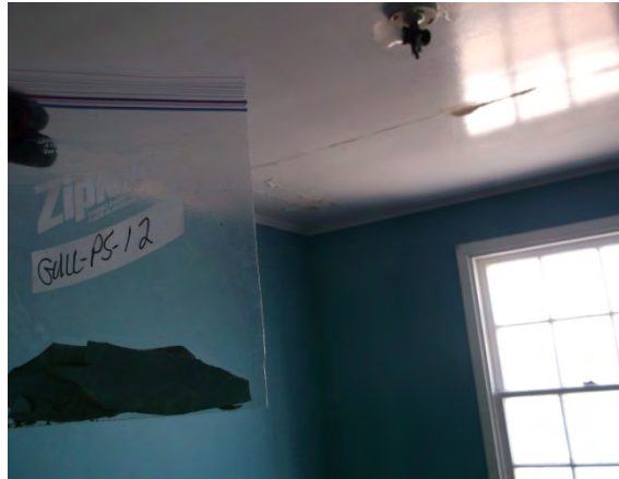
Photo 56: View of paint sample GULL-PS-12.
