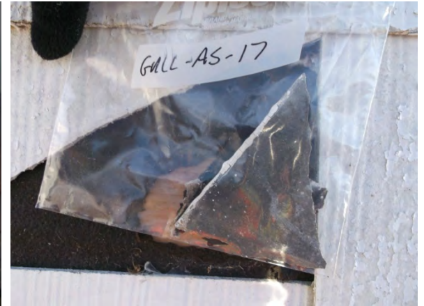
Photo 21: View of cement board siding (transite) sample GULL-AS-17.
