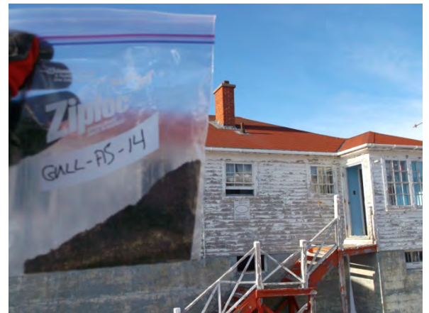
Photo 18: View of asphalt shingle sample GULL-AS-14.
