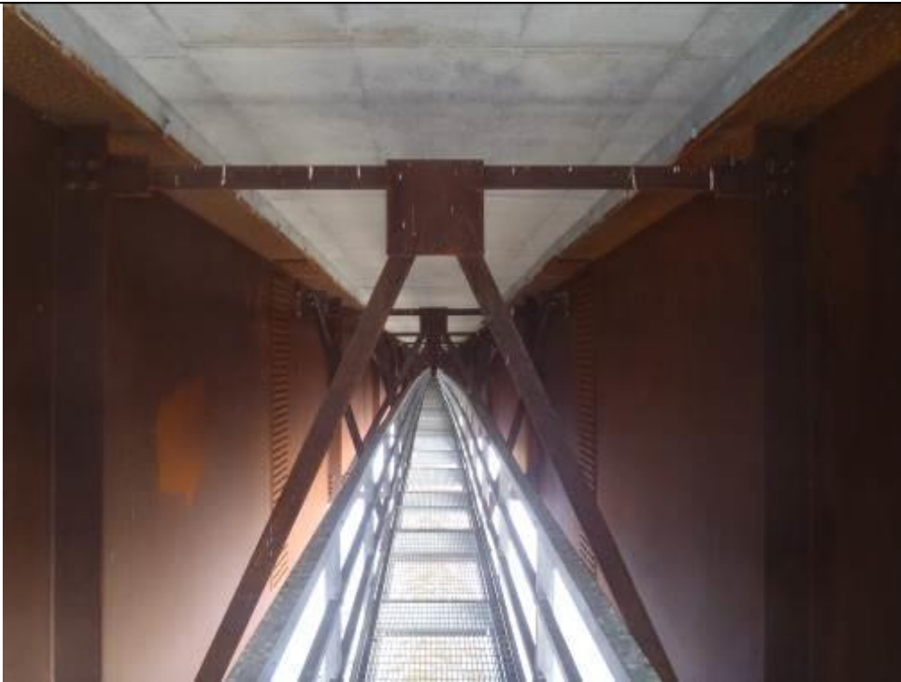
Photo 5 : Girder webs, bracing and catwalk railing
