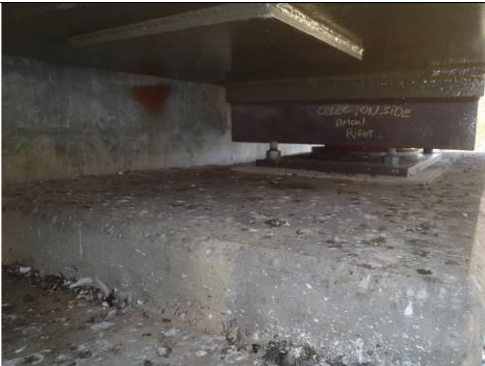
Photo 2 : Abutment seat, below girder
