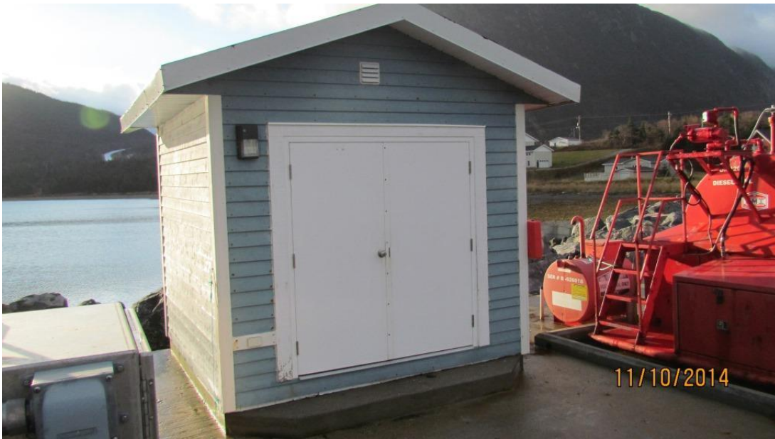
FRC Storage Building (Photo taken 2014)
