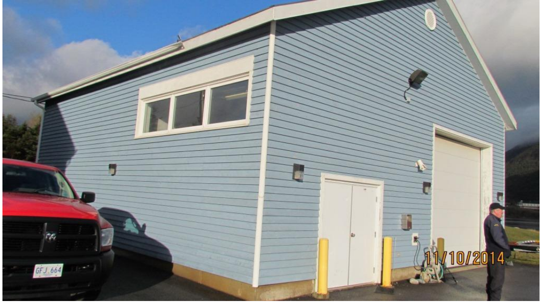
FRC Storage Building (Photo taken 2014)
