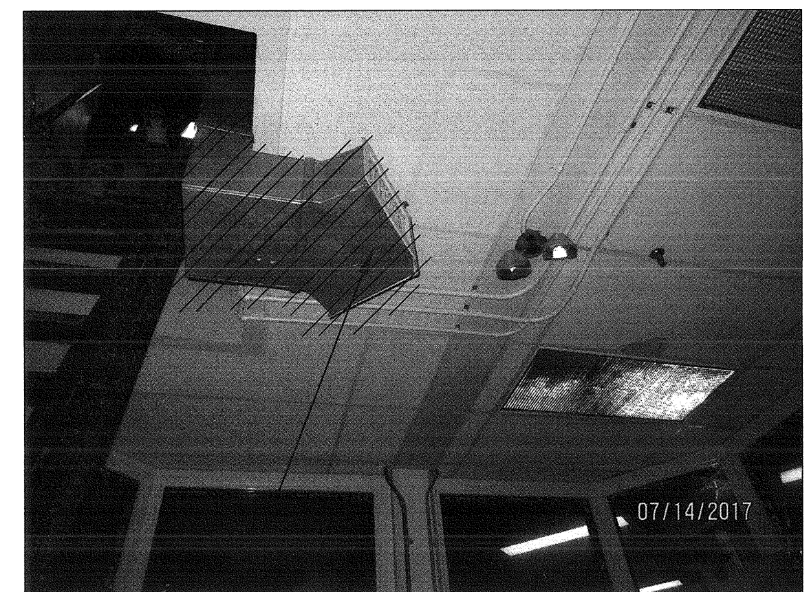
PHOTO-1 DEMOLISH DUCT AND GRILLES
