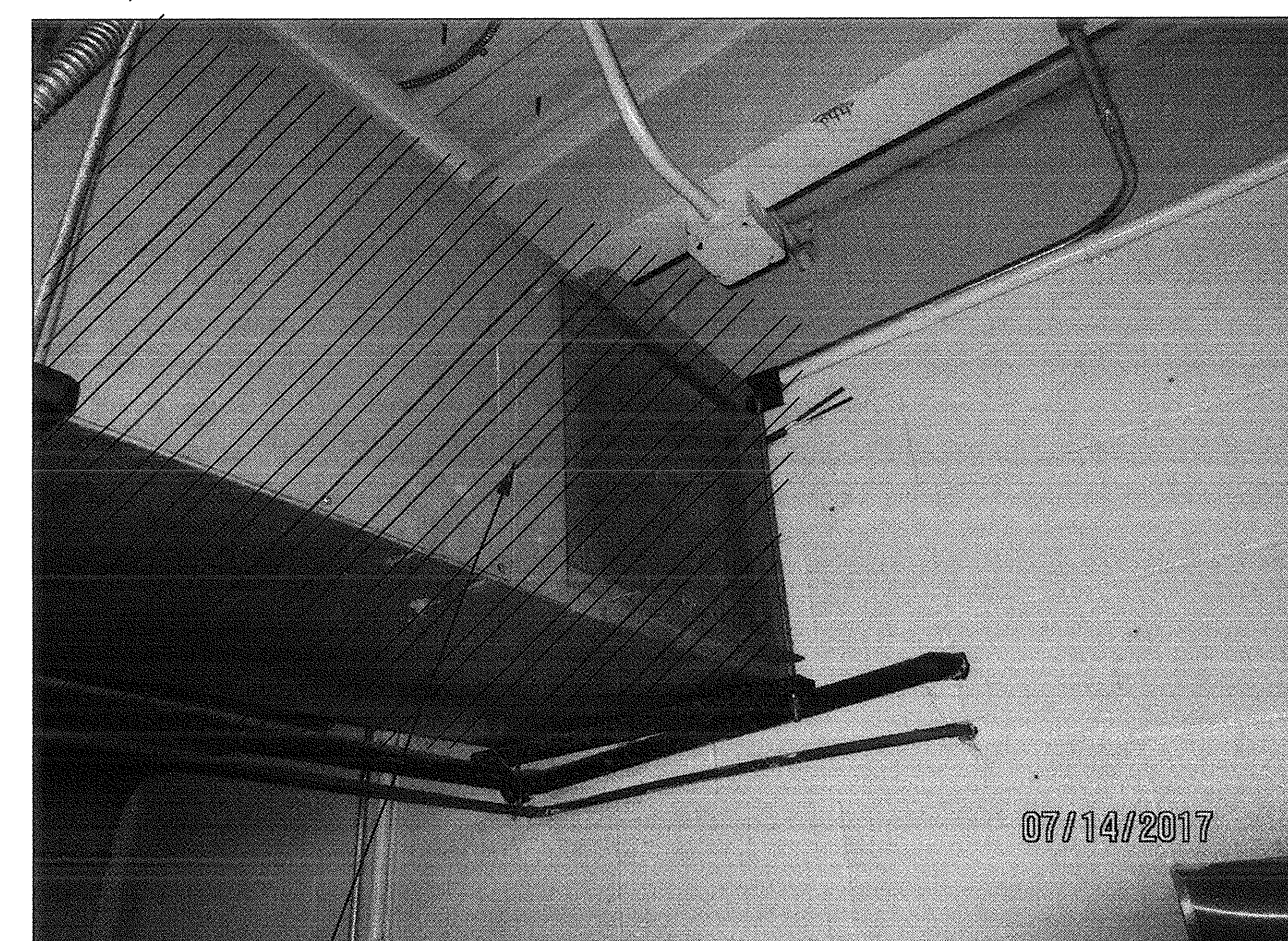
PHOTO-3 DEMOLISH THIS UNIT
