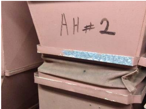
Lead-based "pinkish-brown over beige" paint, Sample L0007.
