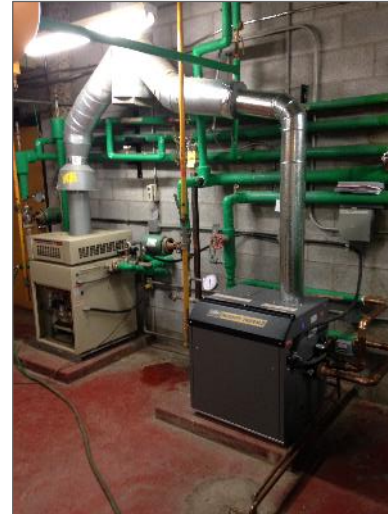
Example of uninsulated mechanical equipment present.
