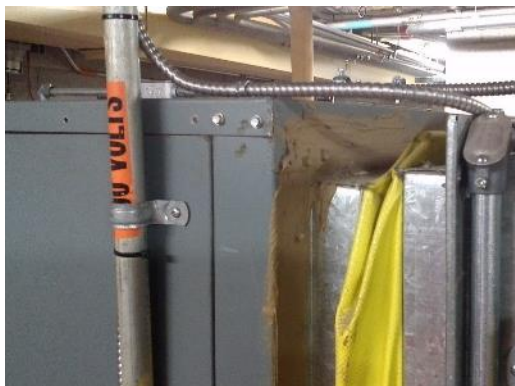
Non-asbestos "brown" mastic, Sample S0008, Southwest Mechanical Room.
