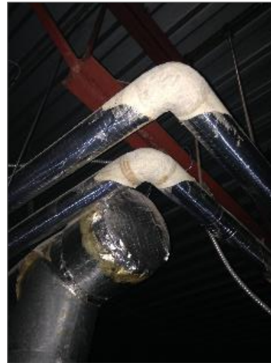
Asbestos pipe elbows in Executive Services
