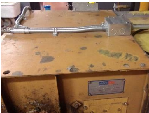
Lead-based "brown" paint, Sample L0003.
