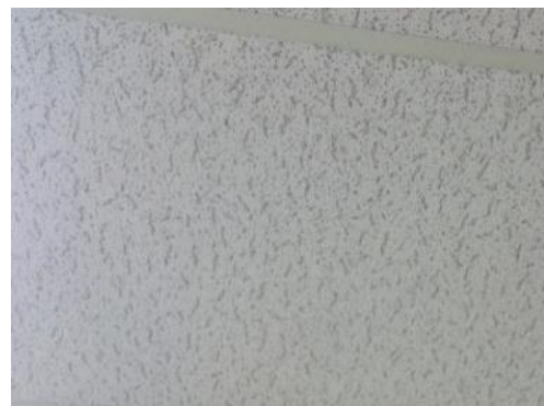
Non-asbestos lay-in ceiling tiles, Sample S0023, Engineering And Maintenance.
