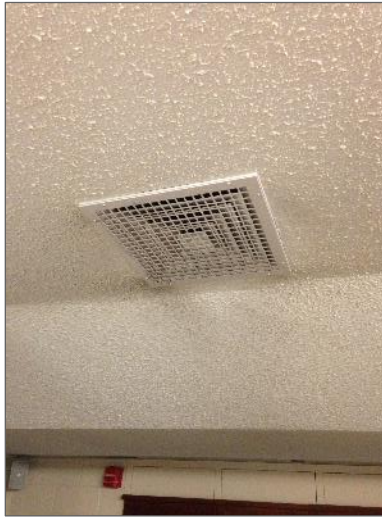
Non-asbestos texture coat present in the Chapel.
