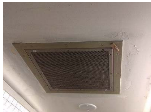
Lead-based "white" paint, Sample L0004.
