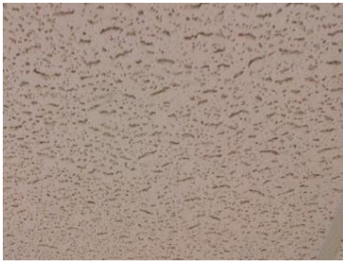
Non-asbestos lay-in ceiling tiles, Sample S0012, Contact Visiting Room.
