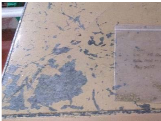
Lead-based "yellow" paint, Sample L0001.
