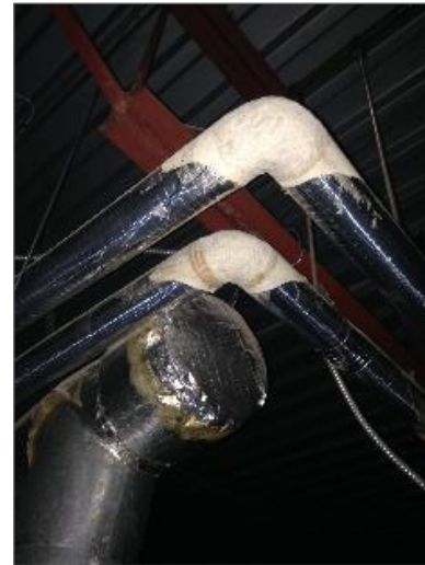
Asbestos pipe elbows in Executive Services
