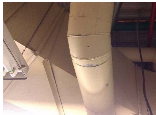
Lead-based "beige" paint, Sample L0006.
