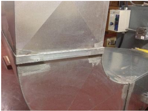
Non-asbestos "silver" mastic, Sample S0006, Southwest Mechanical Room.
