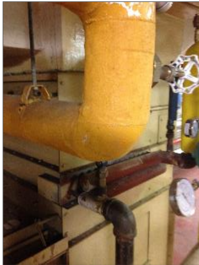
Asbestos pipe elbow in Cell Block Tunnels
