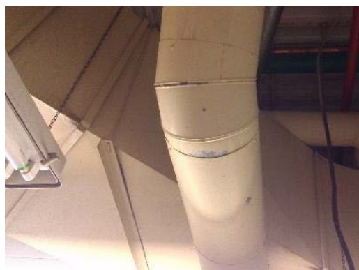
Lead-based "beige" paint, Sample L0006.
