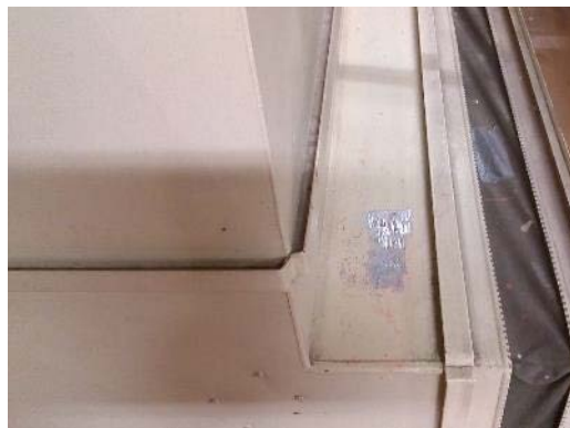
Lead-based "beige" paint, Sample L0002.
