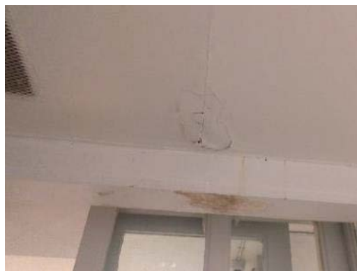
Peeling non-lead based paint in Cell Block A and B office
