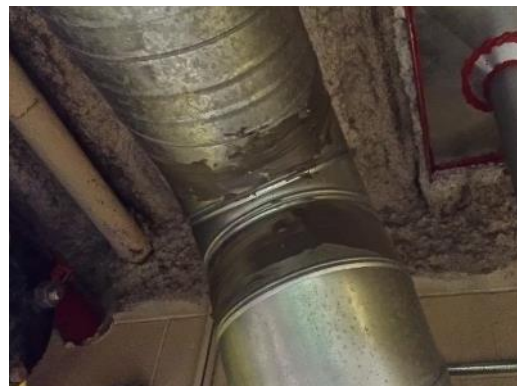
Non-asbestos "grey" mastic, Sample S0016, Segregation Block Mechanical Room.
