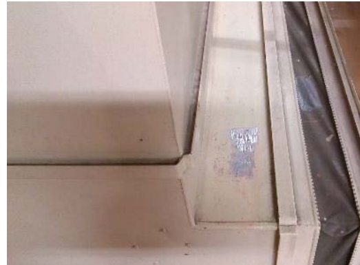
Lead-based "beige" paint, Sample L0002.
