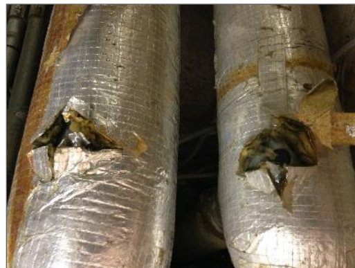
Example of non-asbestos ducting present.
