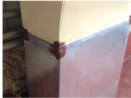
Non-asbestos "red" mastic, Sample S0007, Southwest Mechanical Room.
