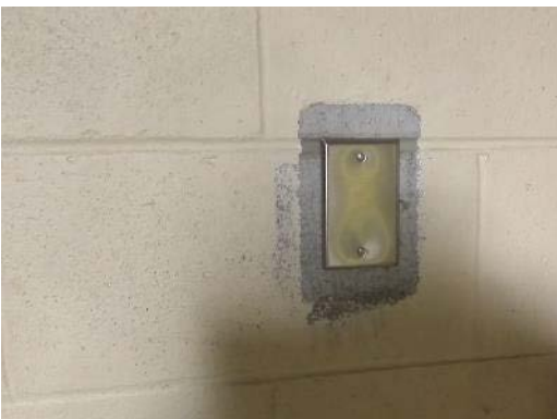
Lead-based "beige" wall paint, Sample L0005.
