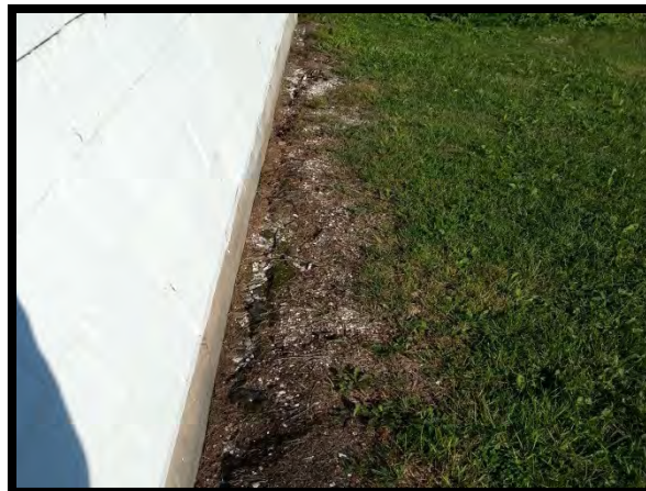
Site (General view of significant weathered exterior white paint – chips on ground)
