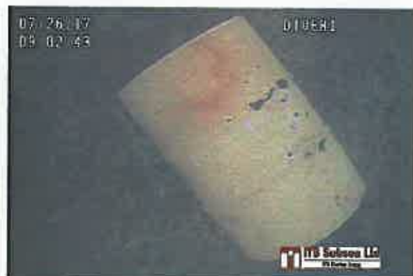
Near e511400, n6663961 obvious corrosion
