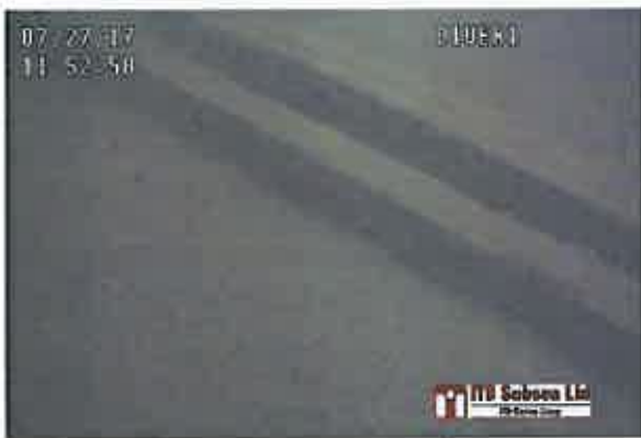
6m timbers with studs, 6m south of #14
