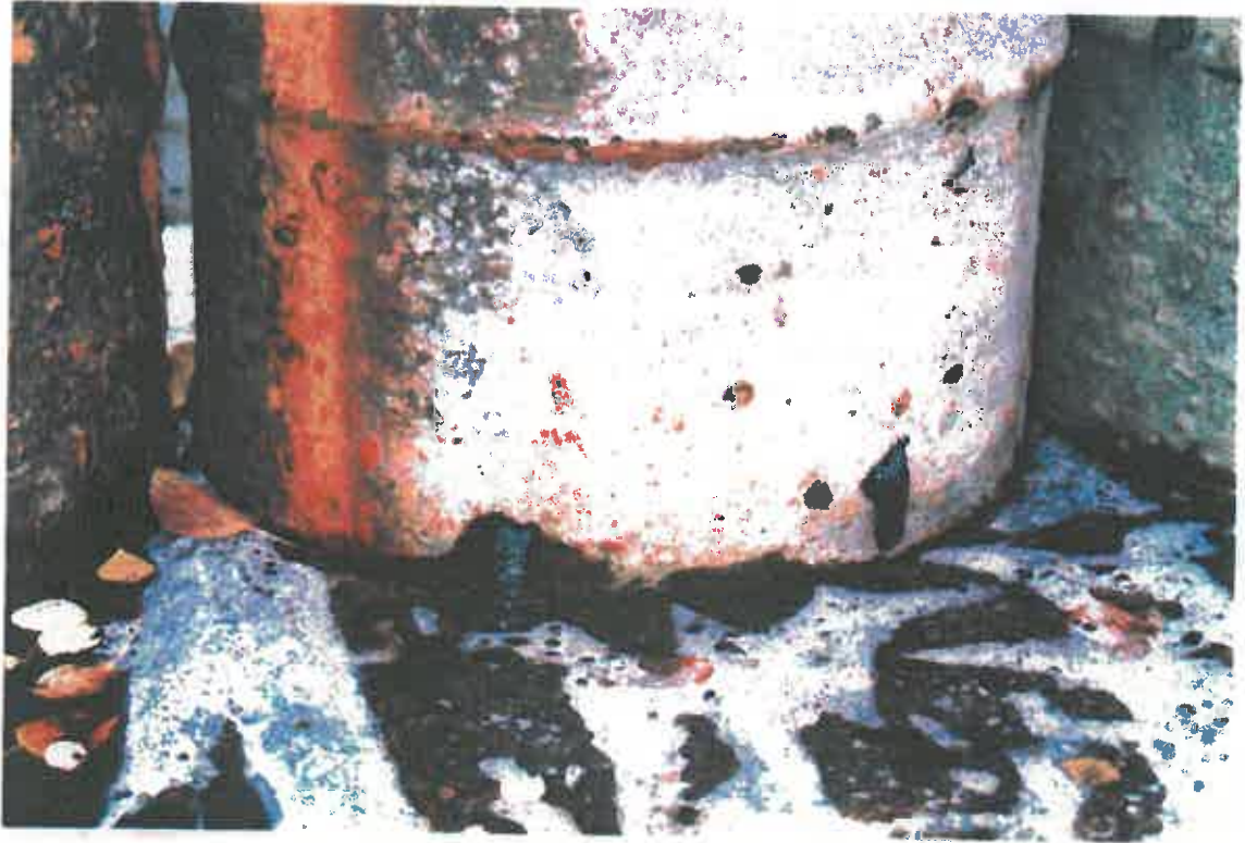
PHOTOGRAPH NO. 17: Black shiny tar-like residue typical of most barrels recovered at the Initial Attack Base. Note higher levels of corrosion damage on the raised rib of the barrel.
